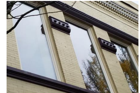
Façade Improvement Project – 313 NE Third Street
