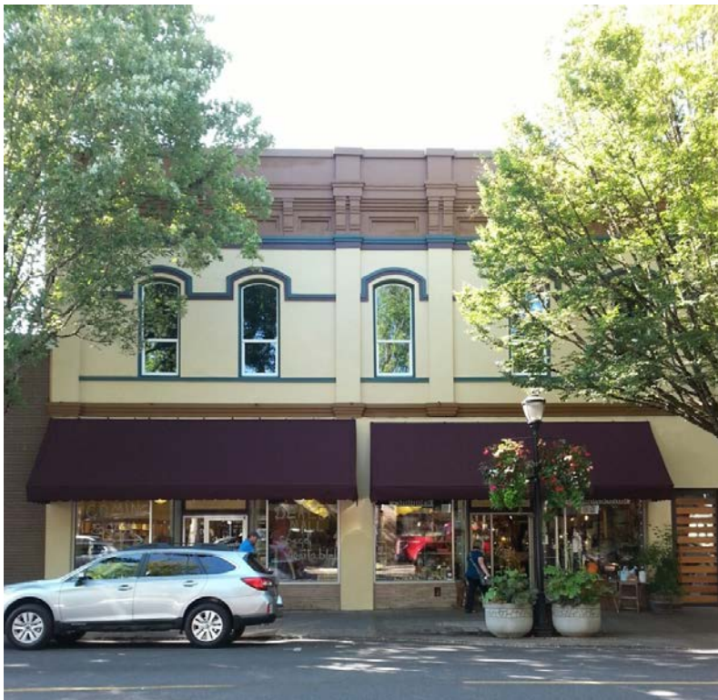
The building had stucco repair, paint and new awnings as part of its façade improvement. (above)
