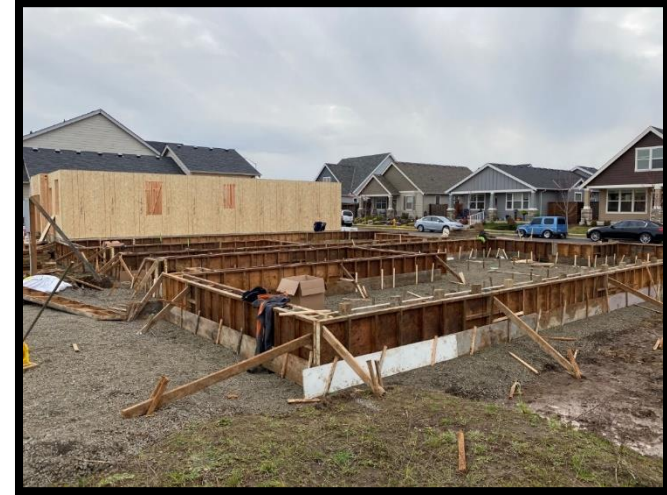
Small Lot, Small Home Subdivision Foundations
