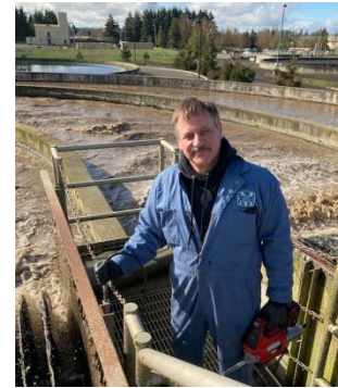
As part of the preventive maintenance program, mechanic David Chitwood, who prefers Joey, is greasing shaft bearings on one of the oxidation ditches.
