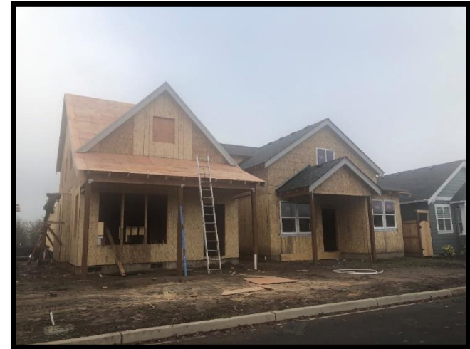
Small Lot, Small Home Subdivision Construction
