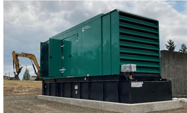
The City continued to invest in upgrades to the public sanitary sewer system in 2021. Work included installation of 1000 KW generators at the Water Reclamation Facility and the Raw Sewage Pump Station.
