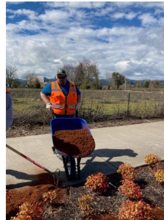
Nick Hubbard - UW II (9mo) spreading bark mulch in Hill Road planters
