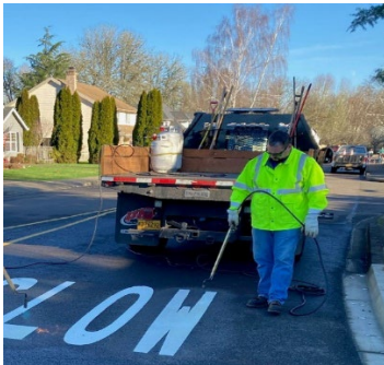
Bud Martino, UW II (2yrs) installing pavement markings on Wallace Road
