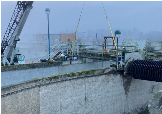
Wastewater Services mechanics guide a shaft as a crane lowers it into place on the oxidation ditch.
