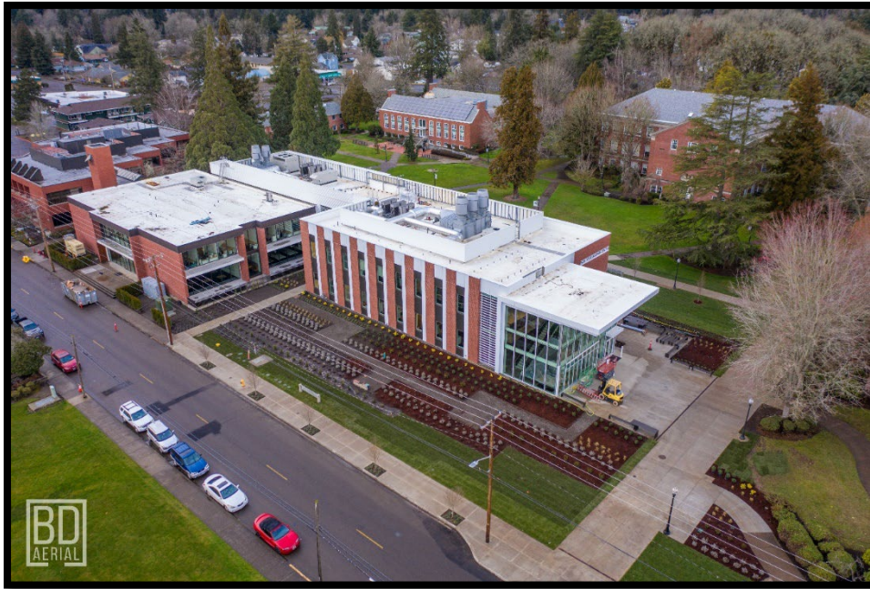
New W.M. Keck Science Building at Linfield University
