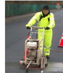
Thermoplastic traffic markings are replaced as necessary, and each stop sign in the system includes a stop bar. Staff replaces approximately 3,100 linear feet (LF) of markings and paints 29,000 LF of curb each year.
