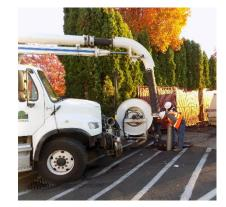
*Conveyance Systems crew cleans a sanitary storm line using one of the City's vacuum trucks.*
