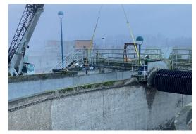
Wastewater Services mechanics guide a shaft as a crane lowers it into place on the oxidation ditch.
