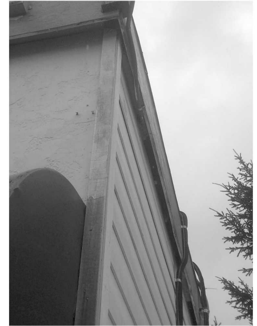
Existing SE corner, note lap siding on east wall of existing wood-framed addition.
