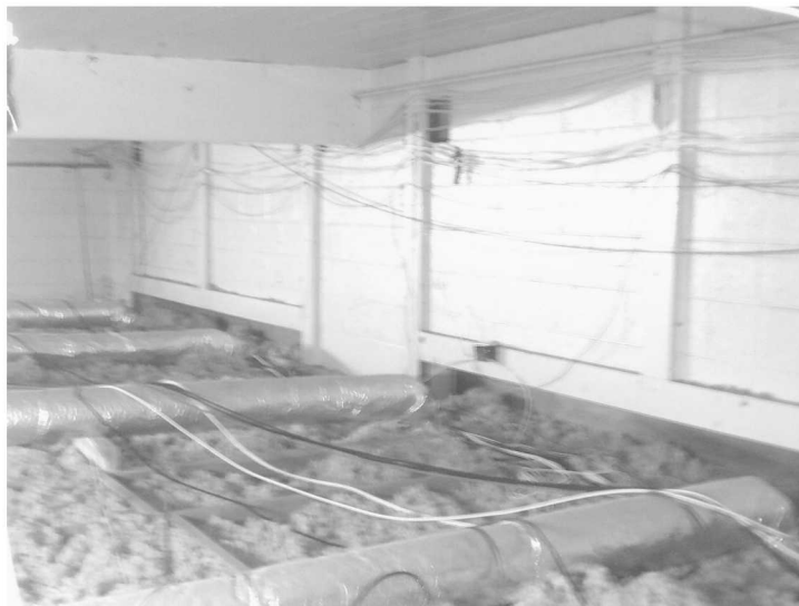
Attic - south wall. Note GLB bears on CMU, between 2 original openings of overhead doors. Note roof decking above, below is ceiling framing with batt insulation and HVAC ducts.
