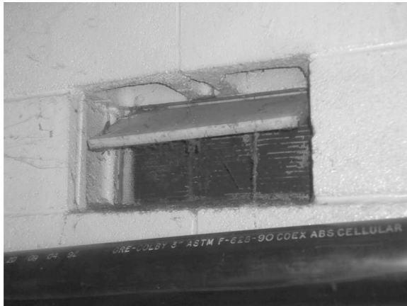
Existing north exterior CMU wall, attic vent in CMU gap. Note CMU above has no grout. Vents are typically dirty.
