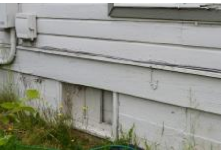
Dry rot to exterior, holes in foundation
