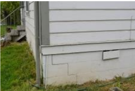
Foundation cracks and separation from the building
