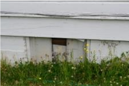
Dry rot to exterior, holes in foundation
