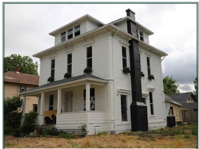
436 SE Baker Street (ca. 1870), Italianate house.
