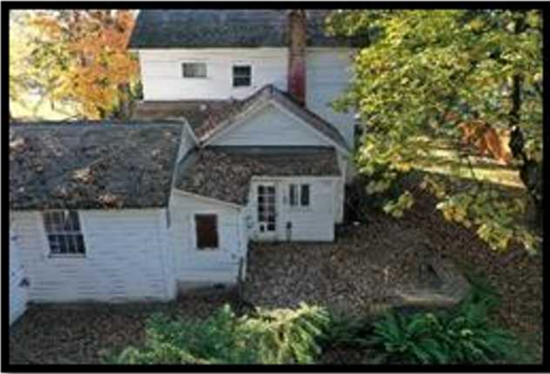
Figure 8: Current view of house and chimney from East
