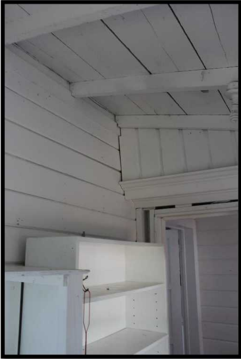
Figure 2: View from within porch addition. Note exterior siding (left) on interior wall
