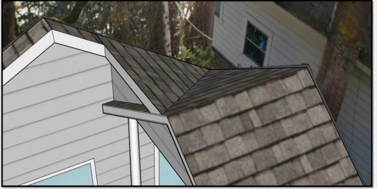
Figure 12: View from above of new roof line and valley
