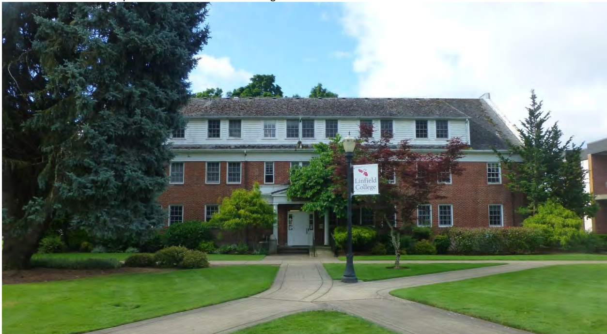
View of north elevation from the academic quad looking south
