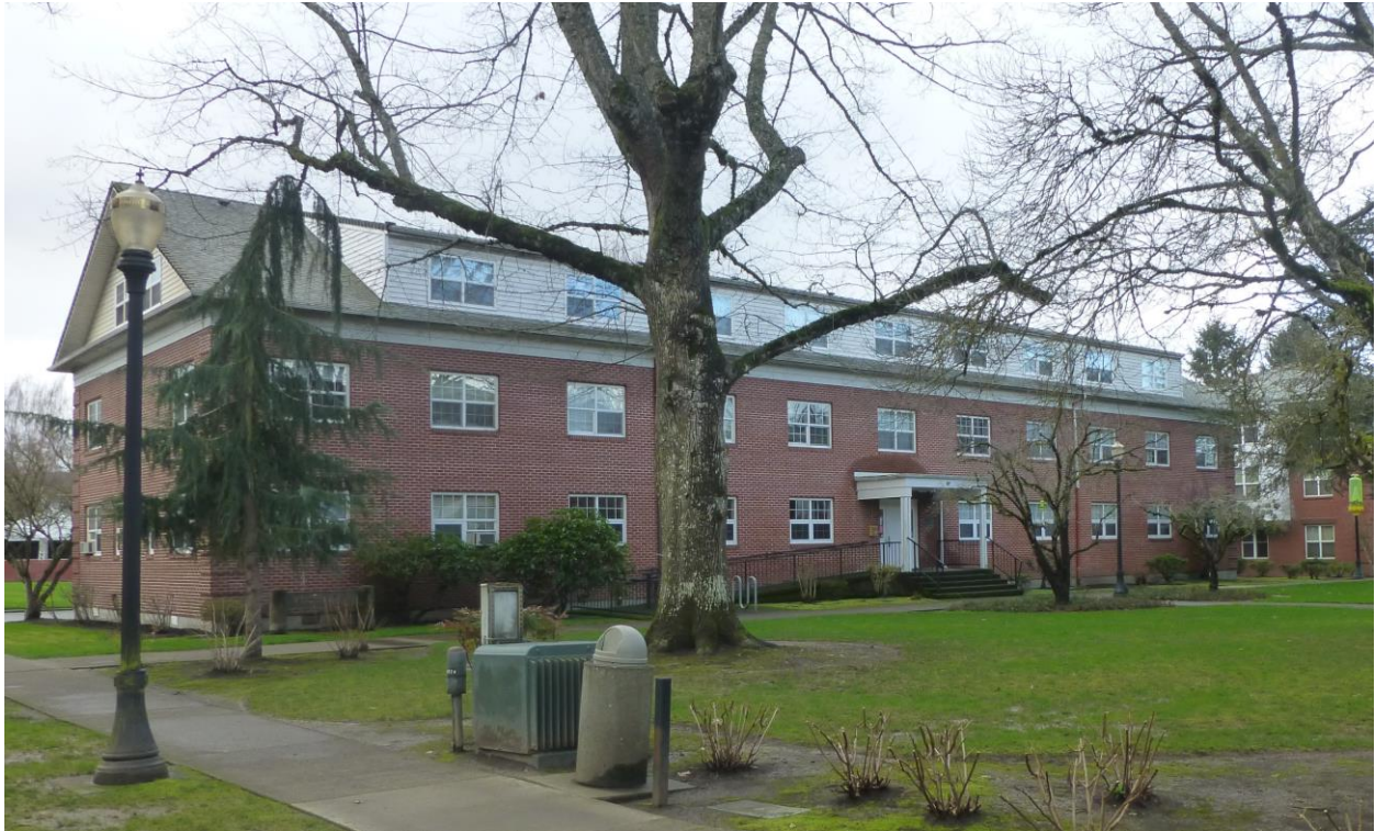
View of south elevation from Linfield Avenue looking to the northwest
