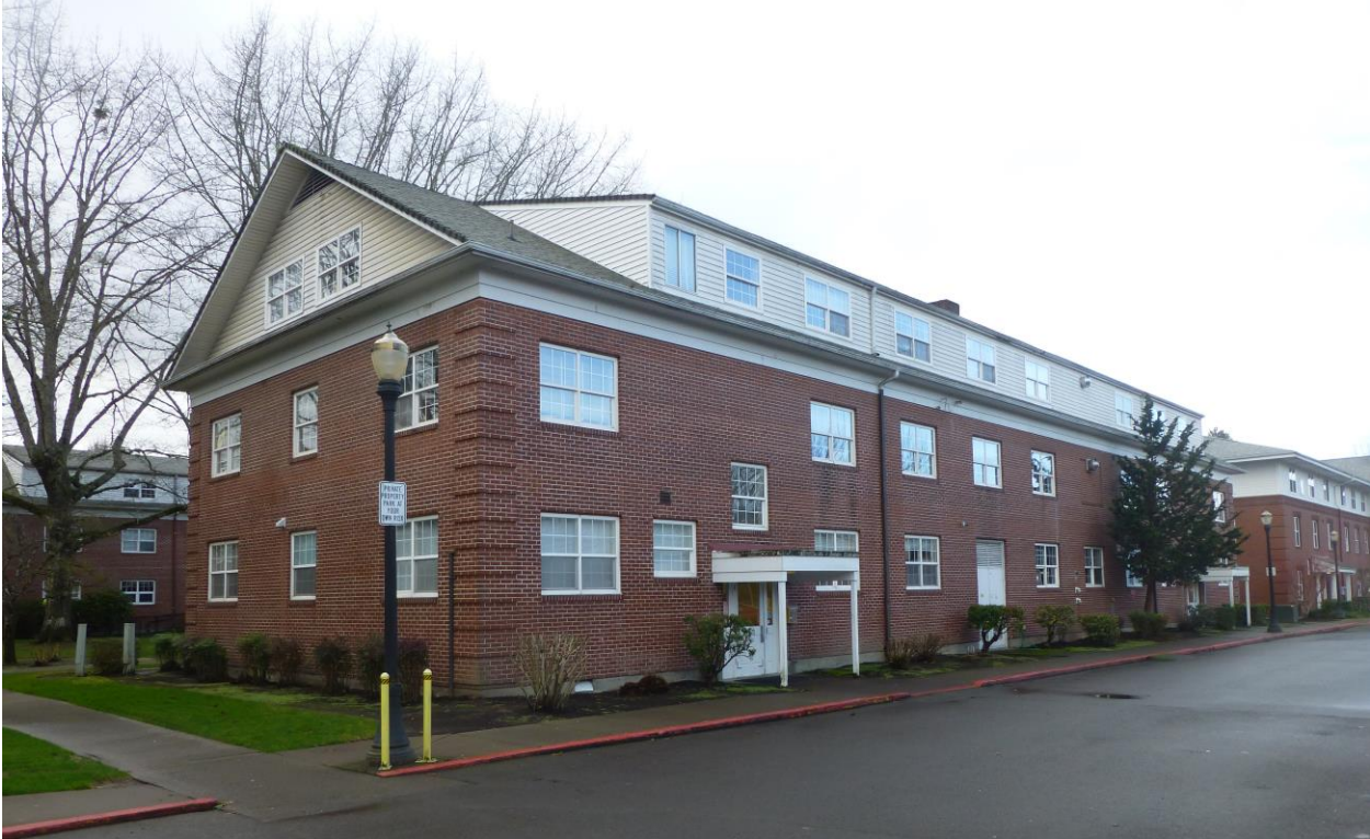
View of northeast elevation
