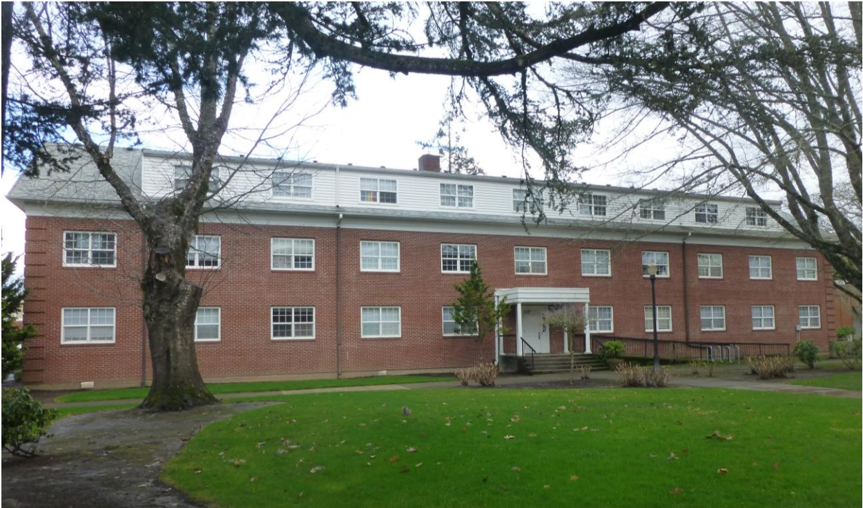
View of south elevation
