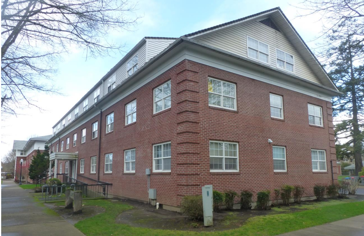
Detail view of northwest elevation
