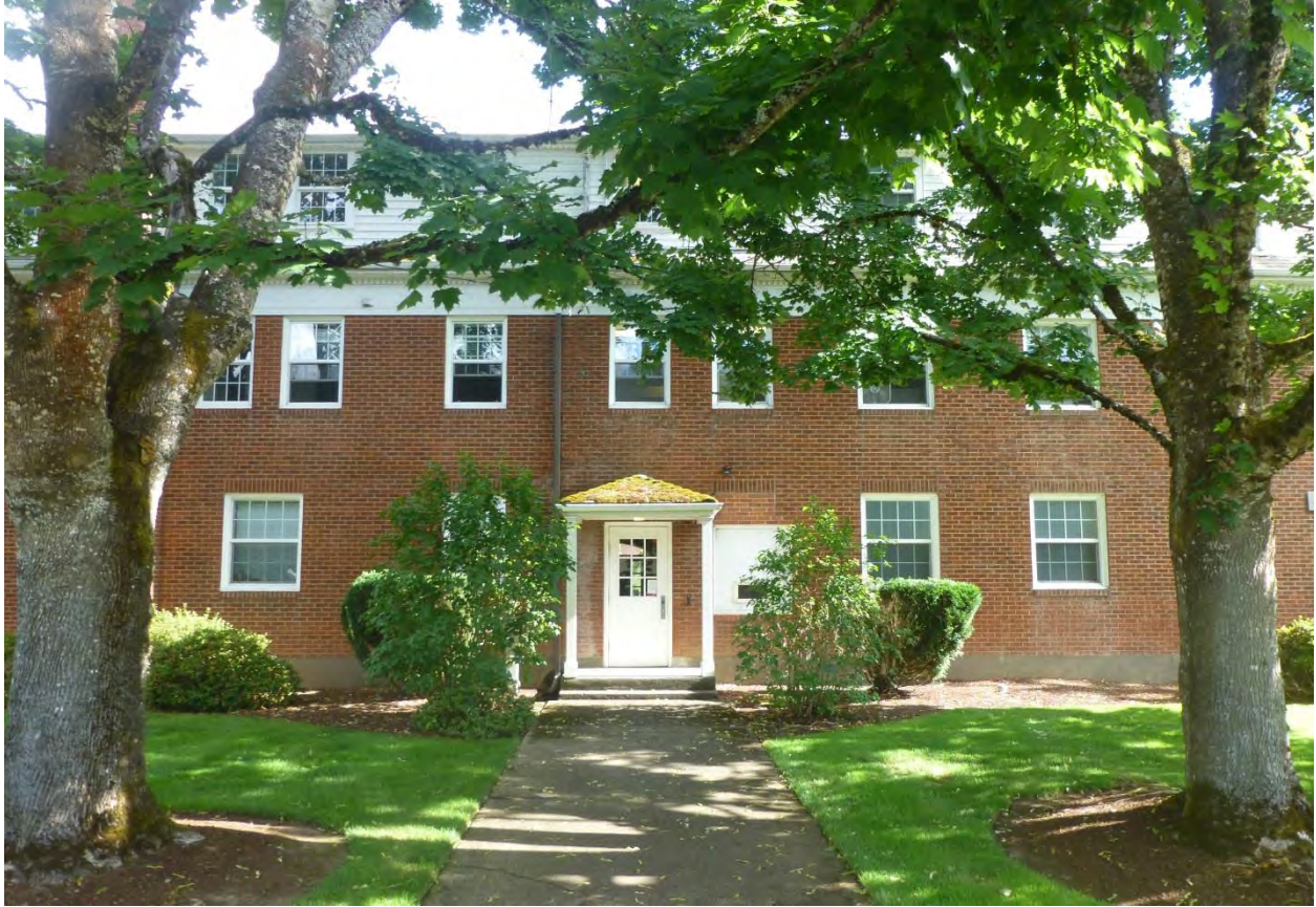
View of south elevation from Linfield Avenue
