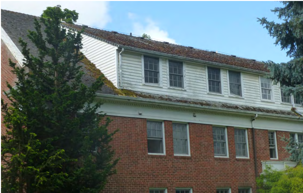
View of northeast building showing roof and siding condition
