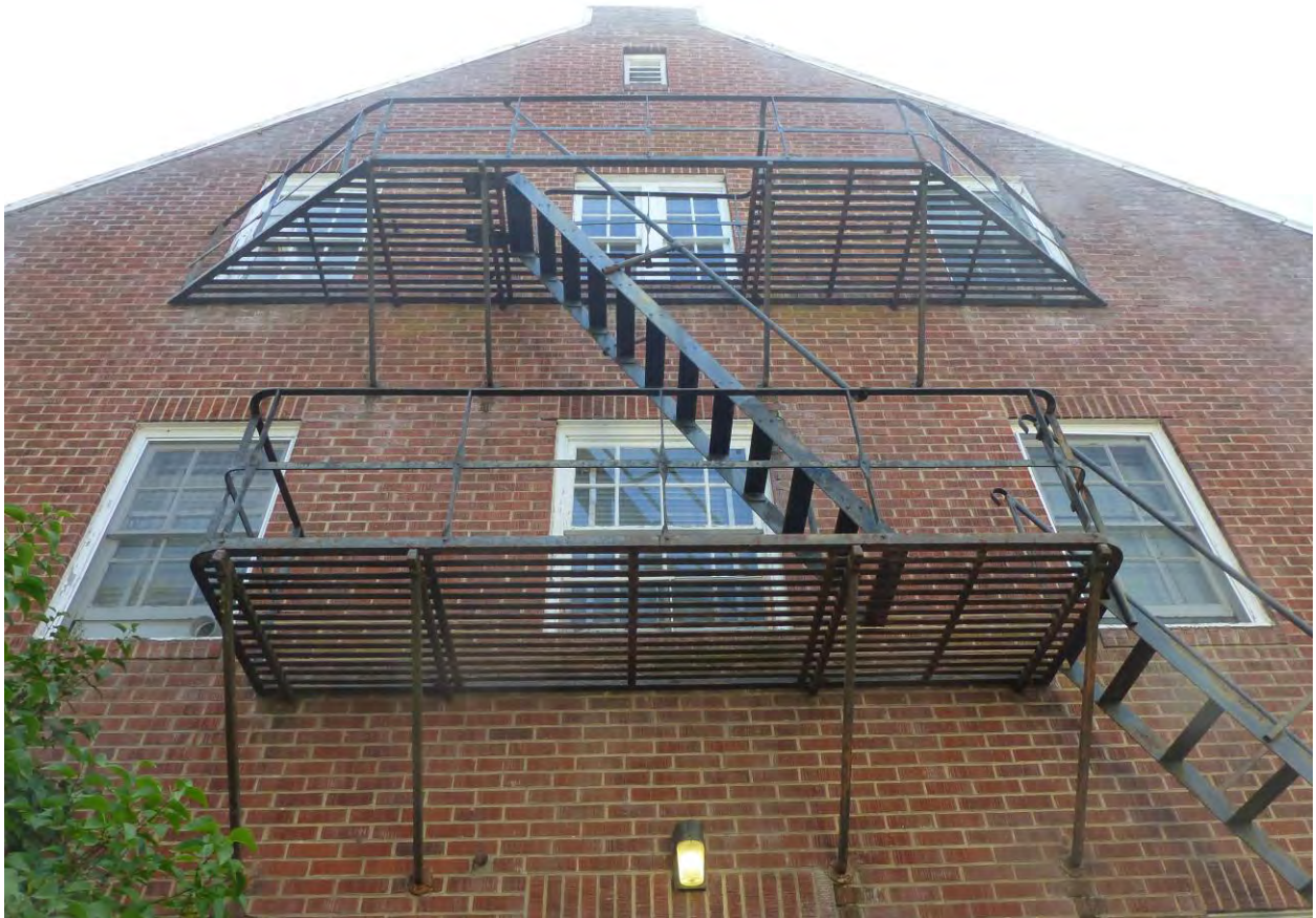
Showing one of two exterior fire escapes.
