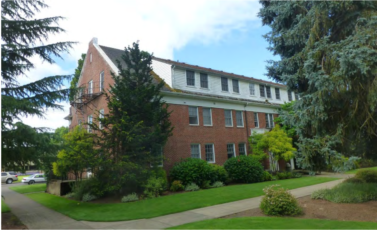
View of north elevation from the academic quad looking south
