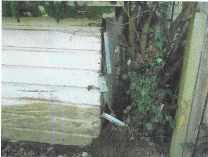
Extensive dry rot, siding was not properly maintained, moisture damage
