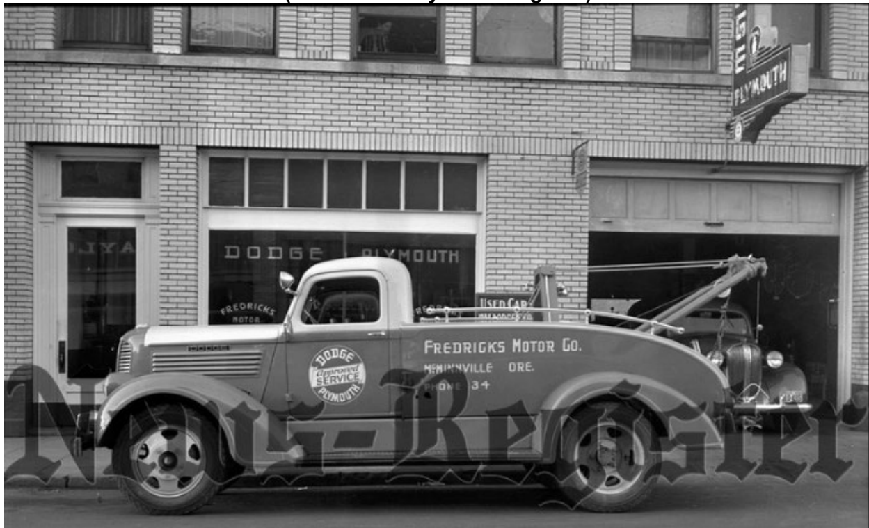
1948 Photo of 611 NE Third Street depicting the ground floor storefront with the original brick veneer. (Yamhill County News Register)
