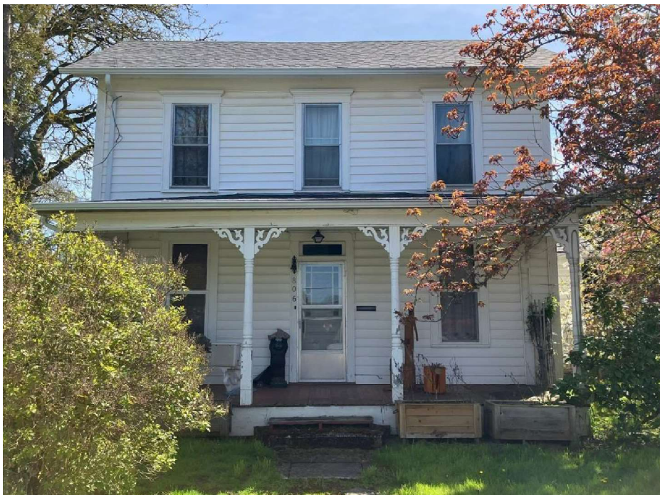
View from Hembree St facing East. This complete side has vinyl siding. All windows and doors look to be original. Front door and upper windows have exterior aluminum storm windows. Decorative elements seem to be in tact.
