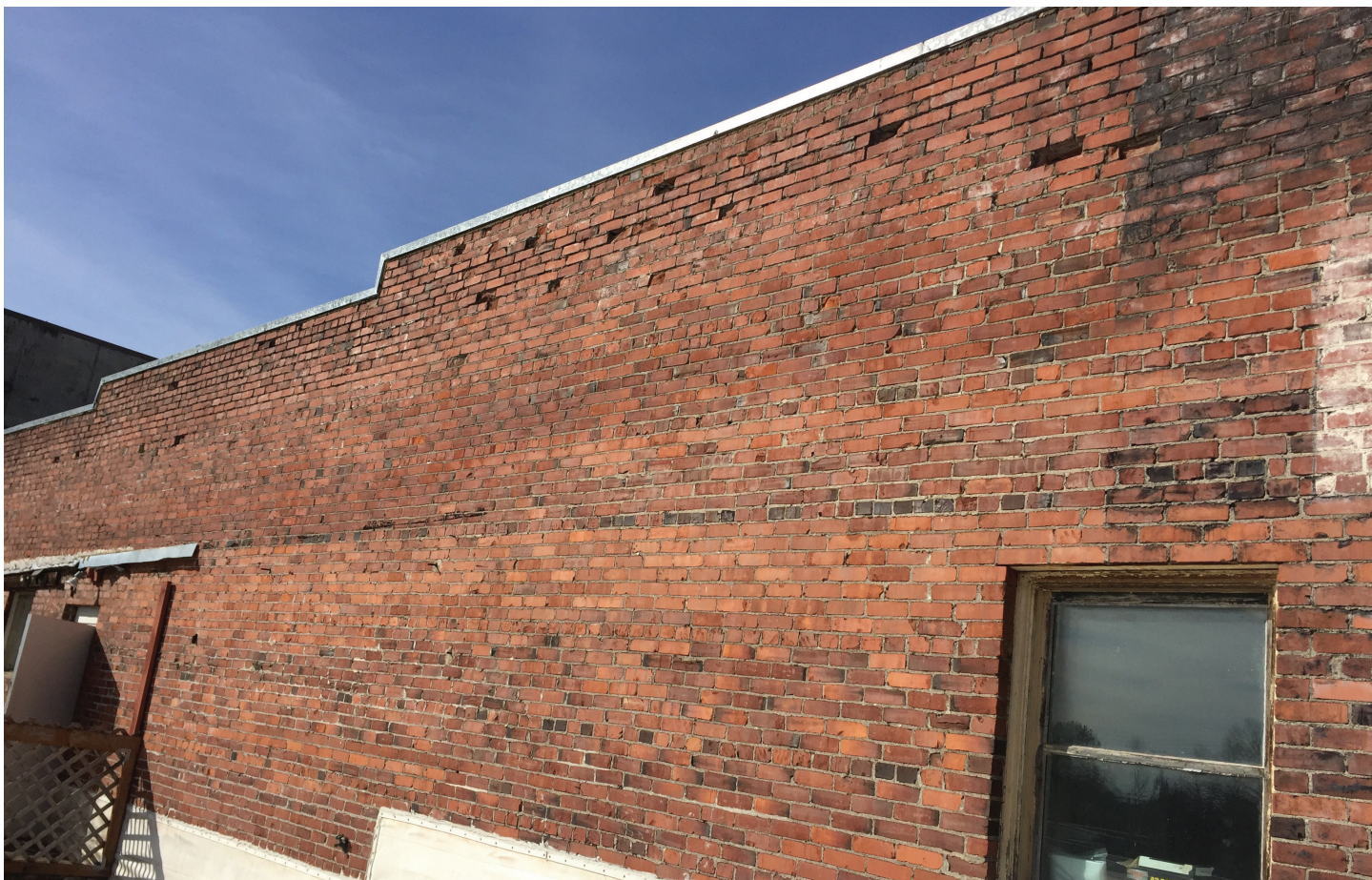
EAST FACADE, SHOWING MISSING AND DAMAGED BRICK
