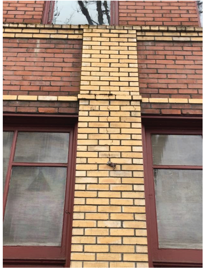
CRACKING IN BUFF-COLORED BRICK AT COLUMNS AND RUSTING OF STEEL LINTELS AT NORTH AND WEST FACADES
