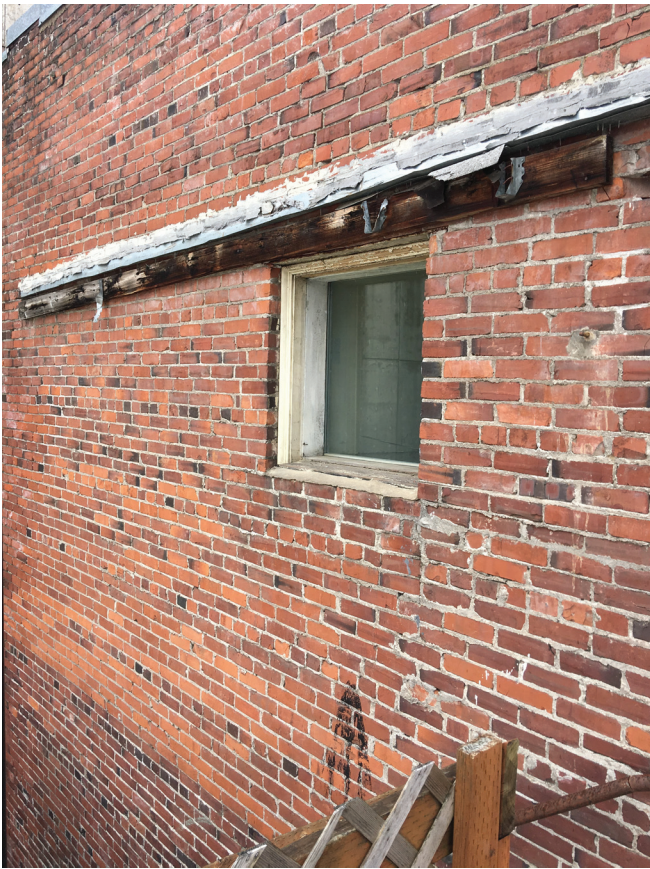
ROOF DECK LEDGER AT EAST FACADE
