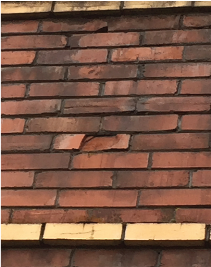
SPALLING BRICK AT WEST FACADE
