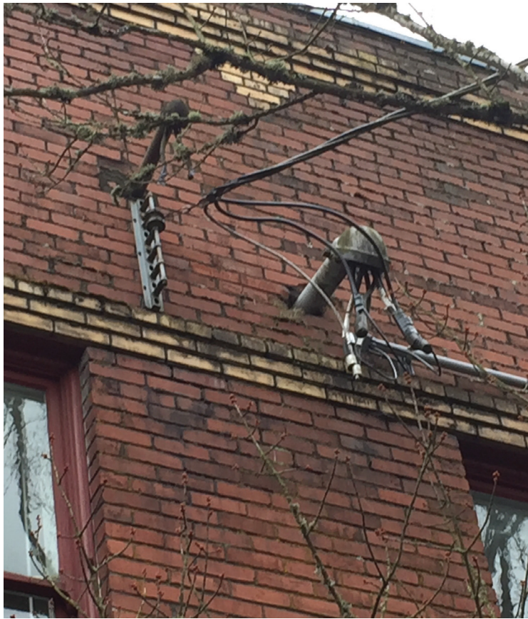
ELECTRICAL SERVICE PENETRATING BRICK
