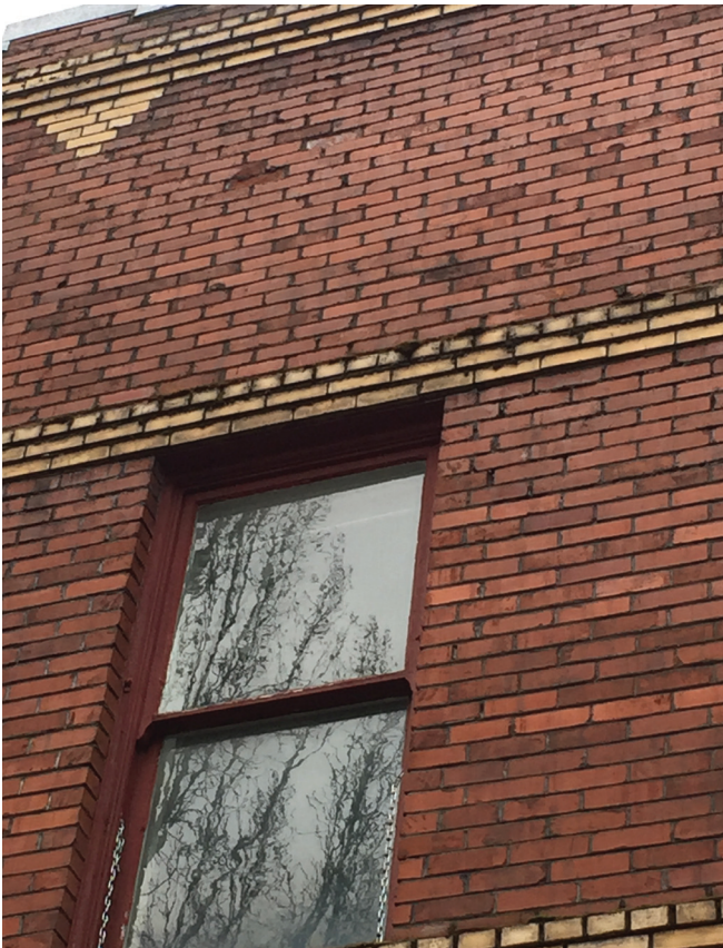
SPALLING BRICK AT WEST FACADE
