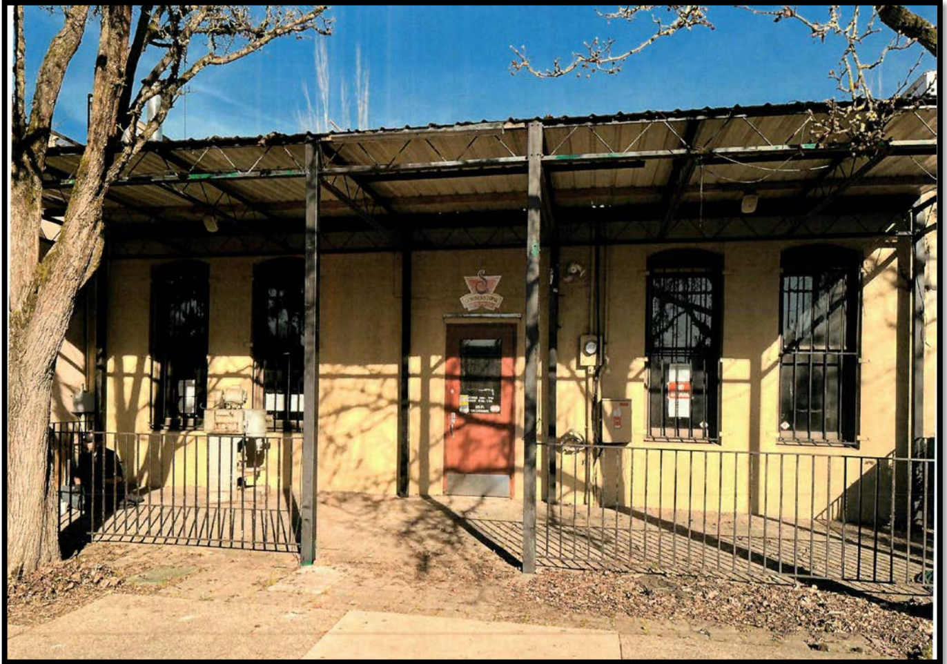
Figure 5. Exterior Photo of Existing Back Facade
