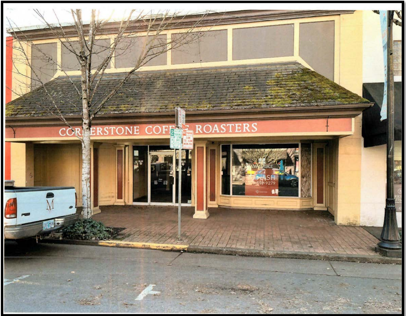
Figure 4. Exterior Photo of Existing Front Facade
