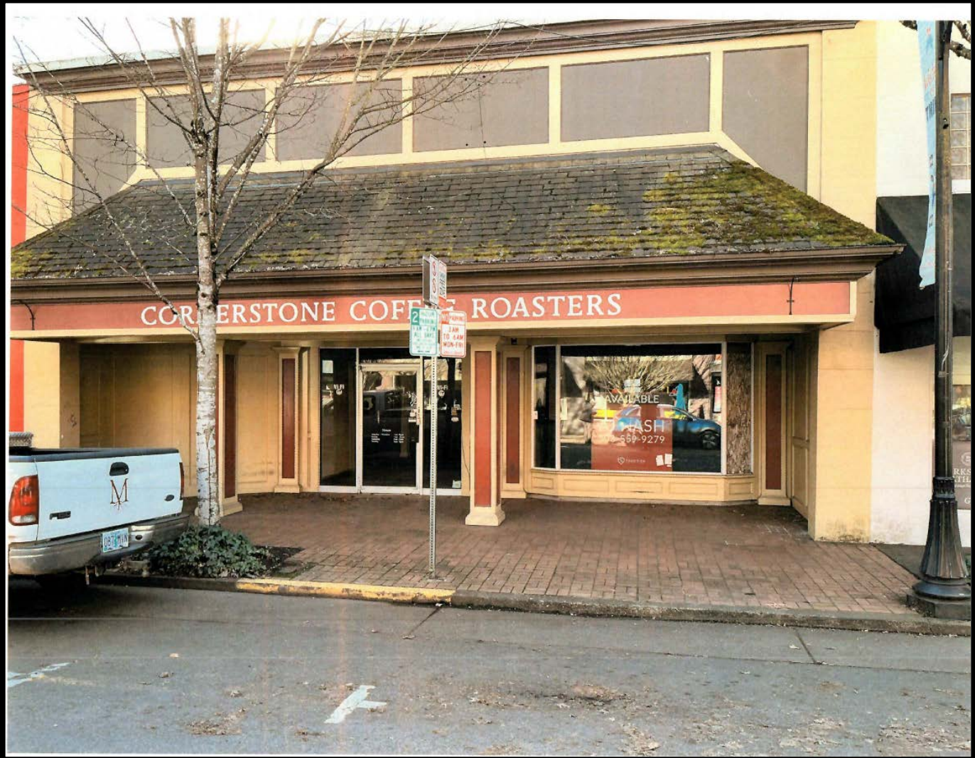
Figure 4. Exterior Photo of Existing Front Facade
