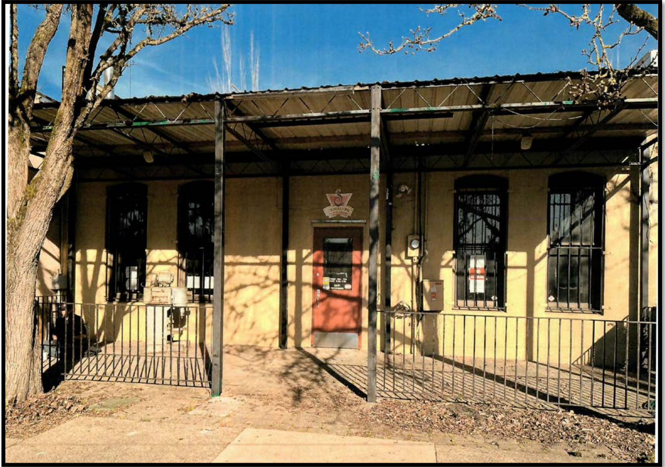
Figure 5. Exterior Photo of Existing Back Facade
