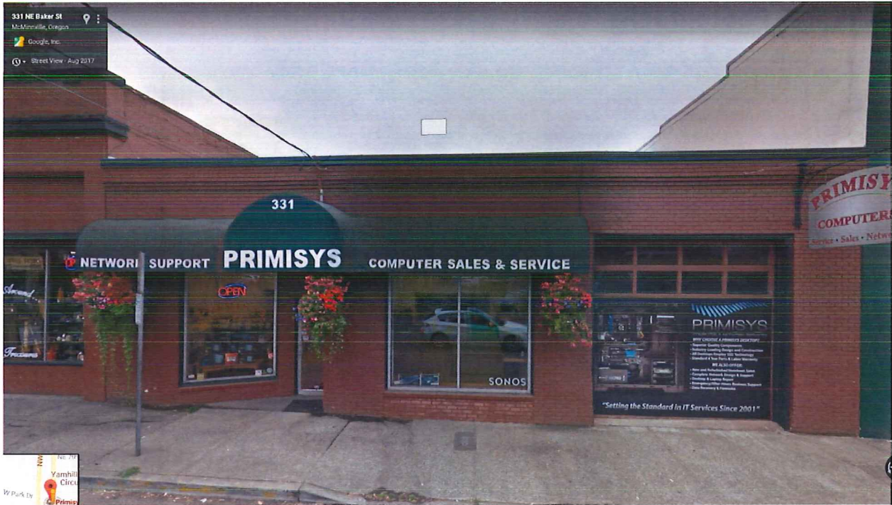
331 NE Baker St aka 337 N Baker Street prior to April 22, 2018 accident
