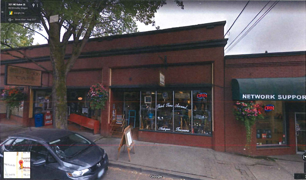
321 NE Baker Street – south of proposed project
