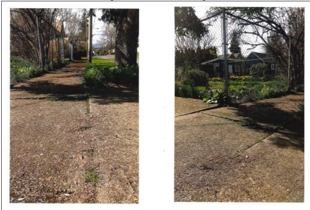
Figure 4: Sidewalk Damage
