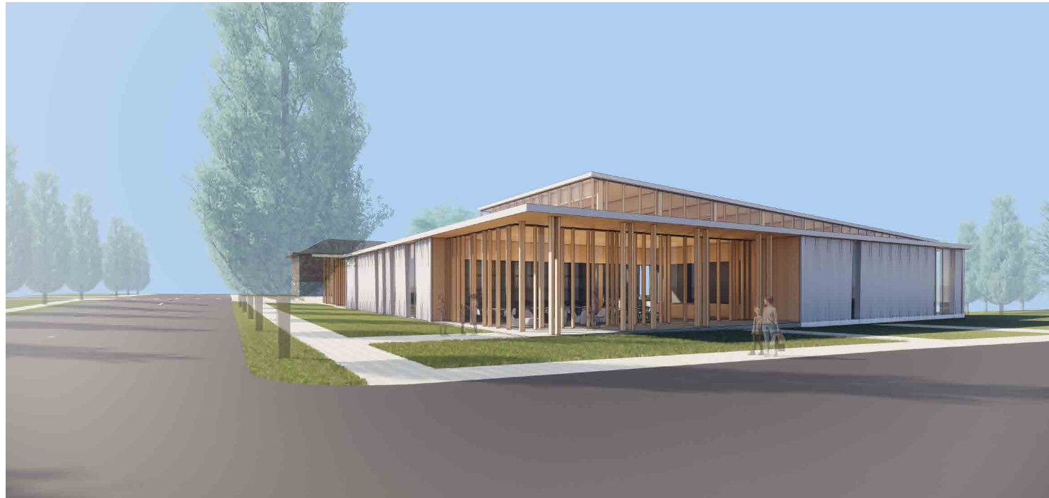
View from 99W and 4th Street of this prominent corner of the library with glass enclosed café style lounge contained within an inviting wood framed loggia with covered bike parking, book-drop and afterhours entrance.
