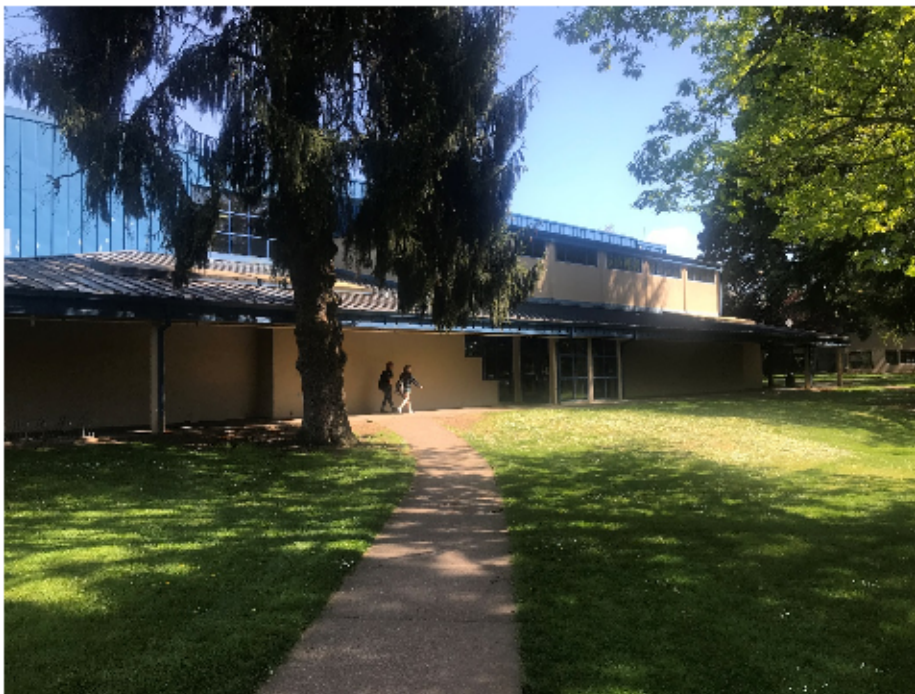
McMinnville Aquatic Center
