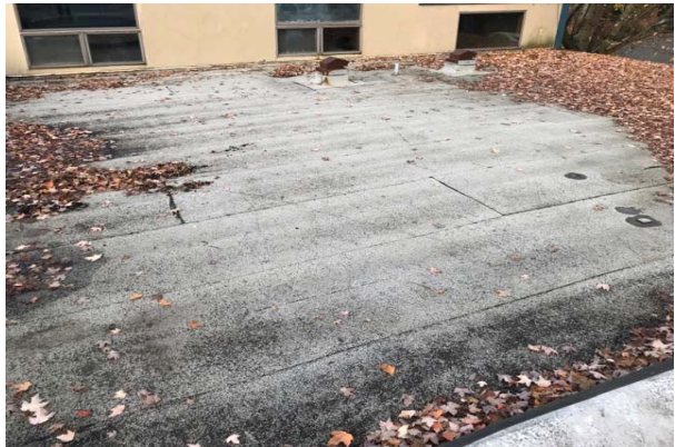
#22 MODIFIED BITUMEN ROOFING
