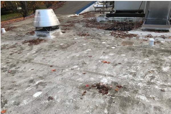
#21 TPO ROOFING MEMBRANE
