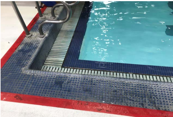
#59 POOL GUTTER SYSTEM
