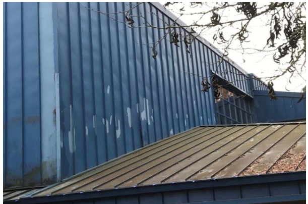
#18 METAL ROOF AND WALL PANELS
