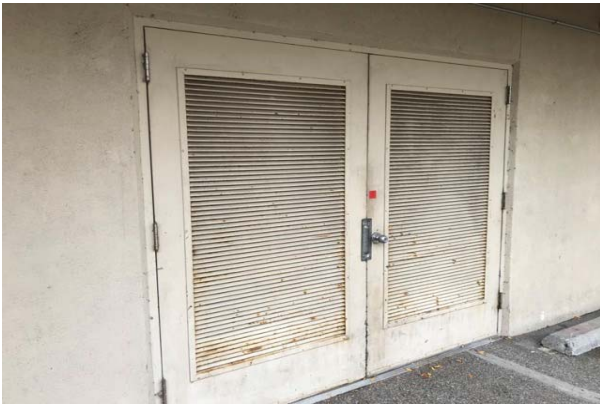
#15 EXTERIOR DOOR, STEEL, REPLACE
