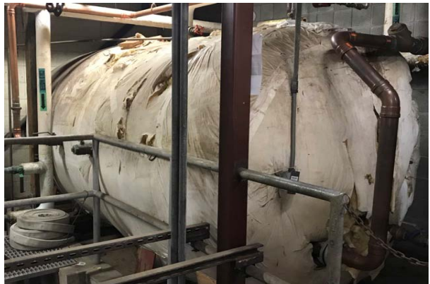
#42 WATER STORAGE TANK
