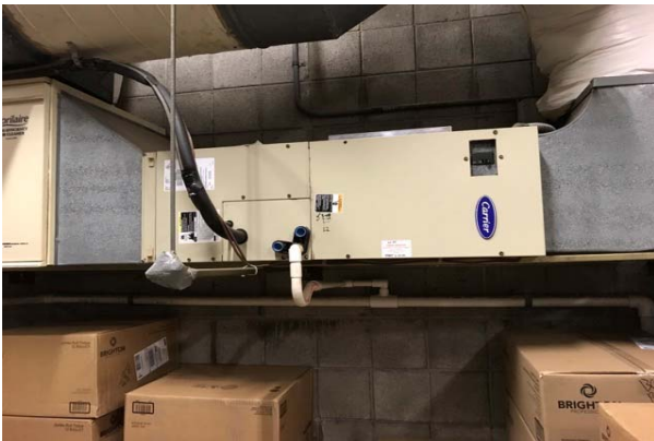
#47 FURNACE, ELECTRIC
