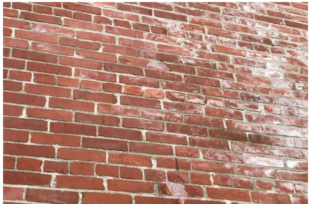
#12 DEGRADED MASONRY
