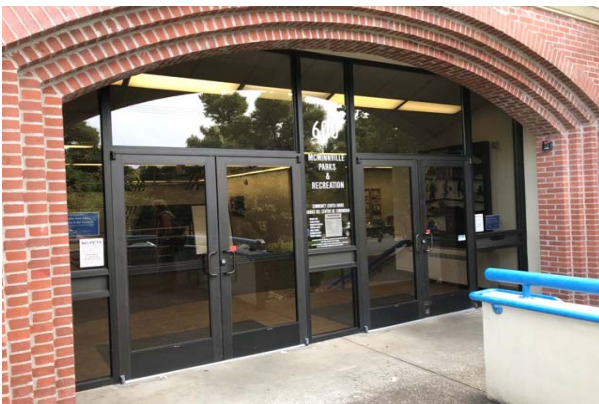
#17 EXTERIOR DOORS, MAIN ENTRANCE
