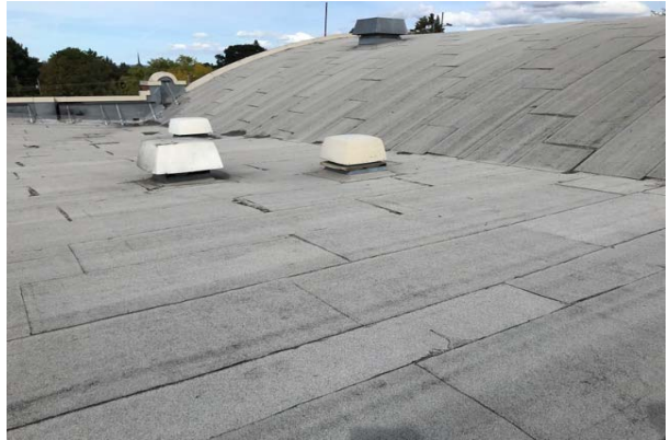
#20 ROOF, MODIFIED BITUMINOUS
