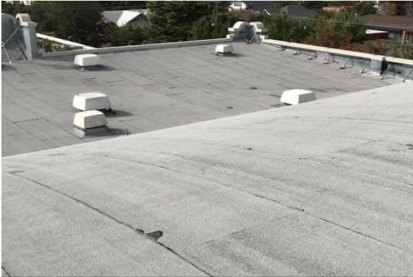
#19 ROOF, MODIFIED BITUMINOUS
