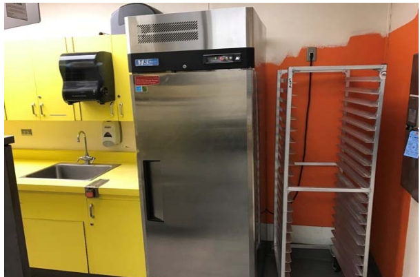
#42 COMMERCIAL KITCHEN, FREEZER
