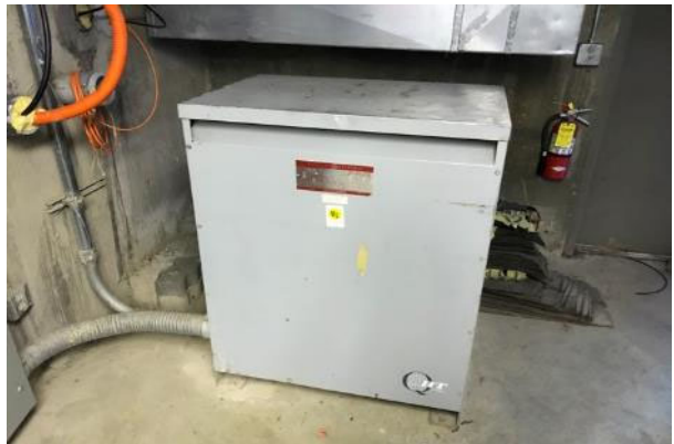
#54 SECONDARY TRANSFORMER
