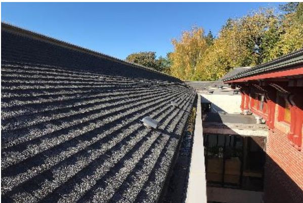
#5 LIBRARY ROOF, ASPHALT SHINGLE
