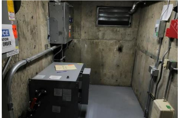
#14 ELEVATOR MACHINE ROOM
