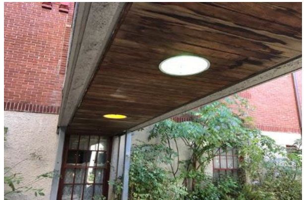
#72 SKY BRIDGE DECKING
