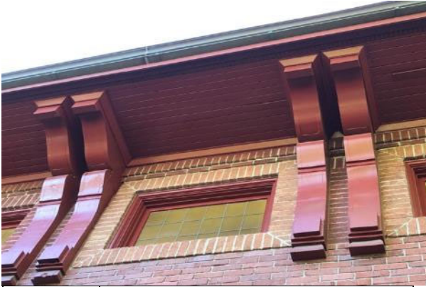
#25 CARNEGIE EXTERIOR WALL
