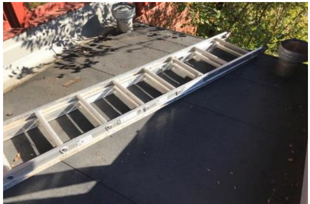
#6 LIBRARY ROOF, MODIFIED BITUMINOUS
