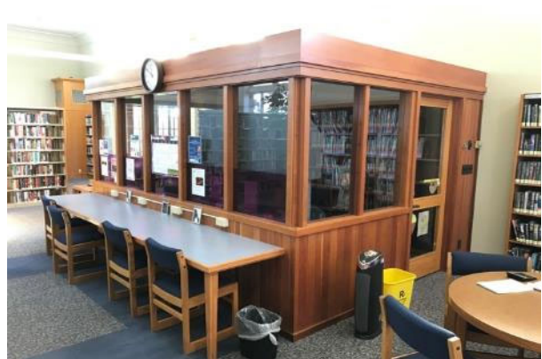
#66 INTERIOR WALL FINISH, WOOD PANELING
