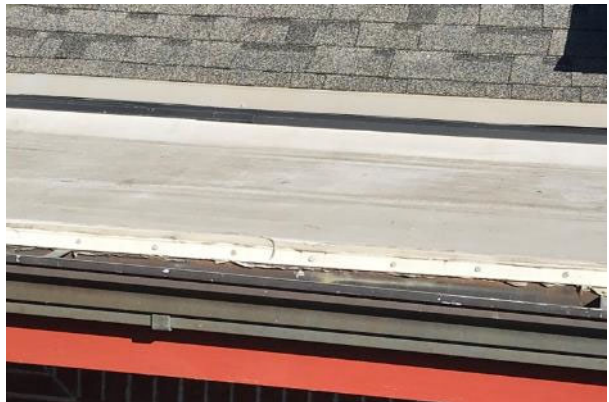
#24 CARNEGIE ROOF, SINGLE-PLY TPO/PVC MEMBRANE
