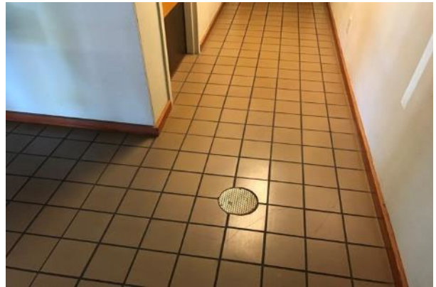
#70 INTERIOR FLOOR FINISH, CERAMIC TILE
