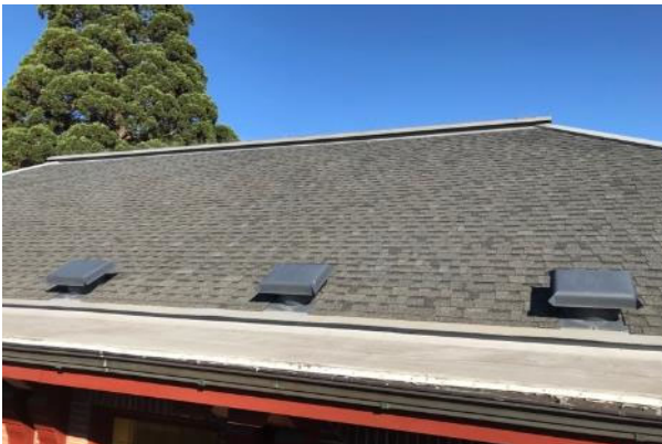
#23 CARNEGIE ROOF, ASPHALT SHINGLE
