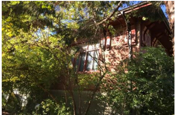
#22 CARNEGIE EAST ELEVATION
