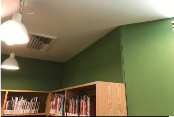
#67 INTERIOR WALL FINISH
