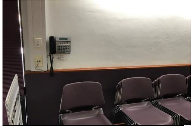
#68 INTERIOR WALL FINISH
