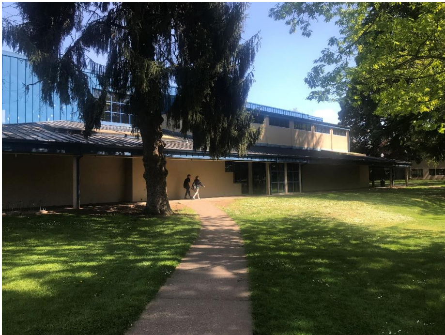
McMinnville Aquatic Center
