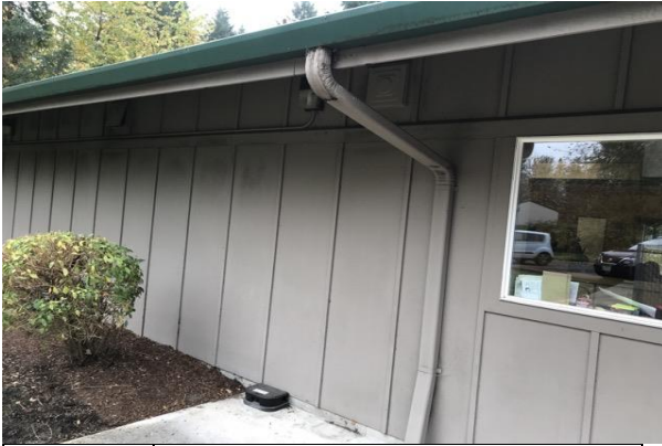
#19 EXTERIOR WALL, GUTTERS AND DOWNSPOUTS
