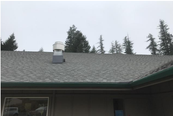
#15 ROOF, ASPHALT SHINGLE
