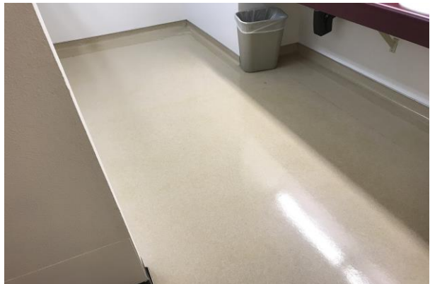
#36 INTERIOR FLOOR FINISH, VINYL SHEET
