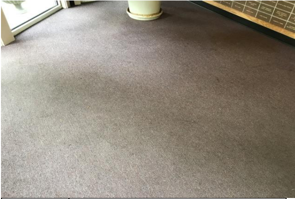
#37 INTERIOR FLOOR FINISH, CARPET
