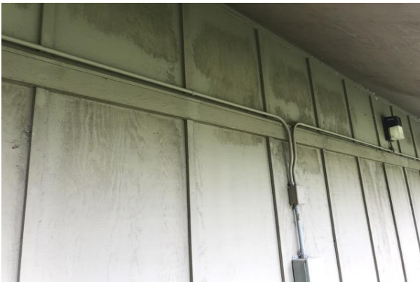
#17 EXTERIOR WALL, PAINTED SURFACE
