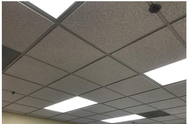
#42 INTERIOR CEILING FINISH, SUSPENDED ACOUSTICAL TILE (ACT)
