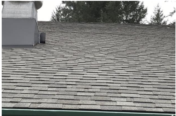
#16 ROOF, ASPHALT SHINGLE
