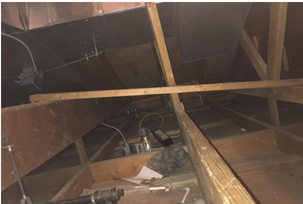
#23 ATTIC, CONVENTIONAL WOOD CONSTRUCTION
