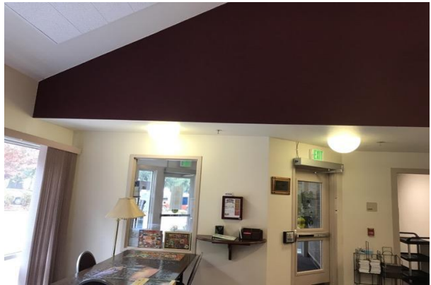
#40 INTERIOR WALL FINISH, GENERIC SURFACE PAINT
