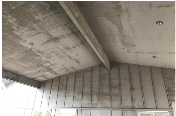
#18 EXTERIOR WALL, PAINTED SURFACE
