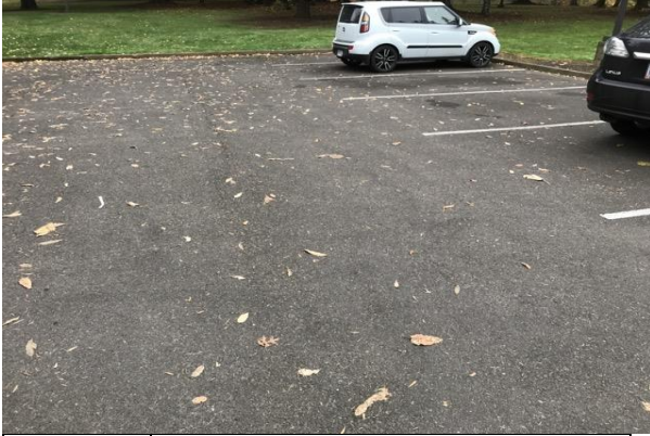
#7 PARKING LOTS, ASPHALT PAVEMENT
