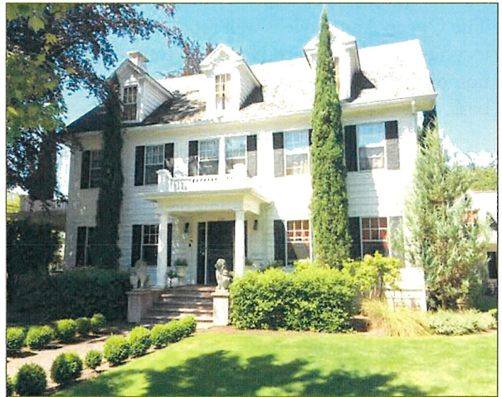
COLONIAL REVIVAL EXAMPLES WITH THE FRANK W. FENTON HOUSE AT 434 NE EVANS STREET (UPPER) AND 809 NE EVANS STREET (LOWER).
