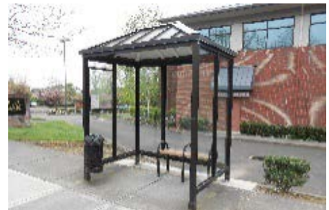
Figure 7-7 Brutscher Street Shelter, Newberg
