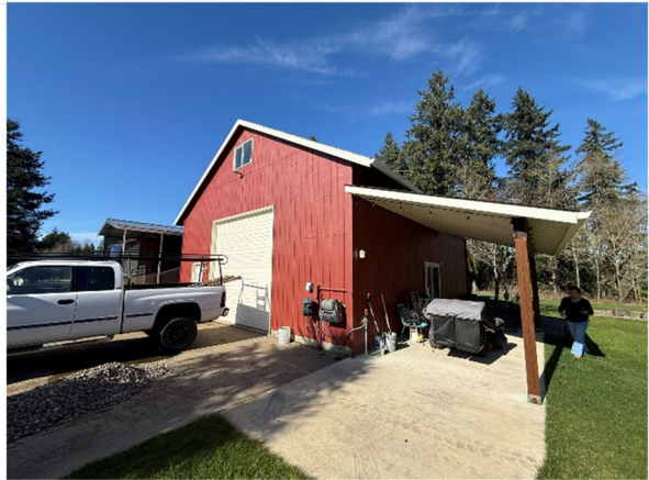
Photo #16 Permitted Shop/ADU on TL 690, facing northwest
