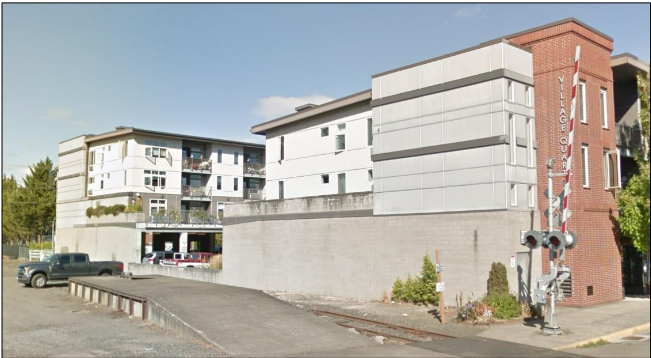
Village Quarter west building façade:
