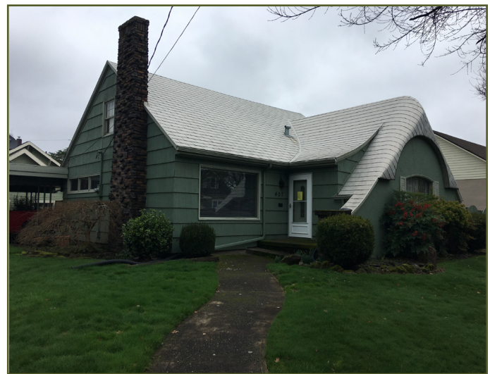
TWO EXAMPLES OF ENGLISH COTTAGES AT 407 NE 12TH STREET (LEFT) AND 540 NW BIRCH STREET (RIGHT).
