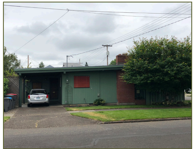
CONTEMPORARY STYLE 405 NE 11TH STREET.
