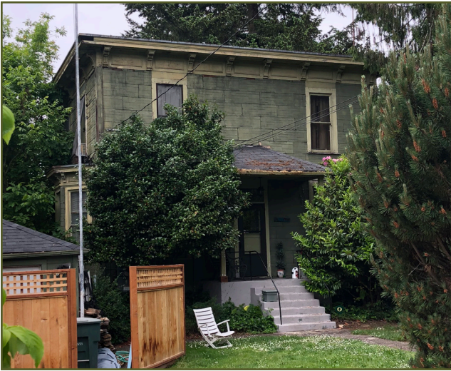
ANDREW JEFFERSON NELSON HOUSE (1875) AT 501 NW BIRCH STREET IS AN EXAMPLE OF A RESIDENTIAL APPLICATION OF THE ITALIANATE STYLE.
