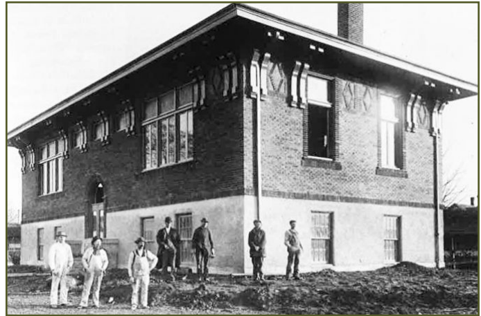
1913 PHOTO OF THE CARNEGIE LIBRARY. COURTESY HISTORIC McMINNVILLE.
