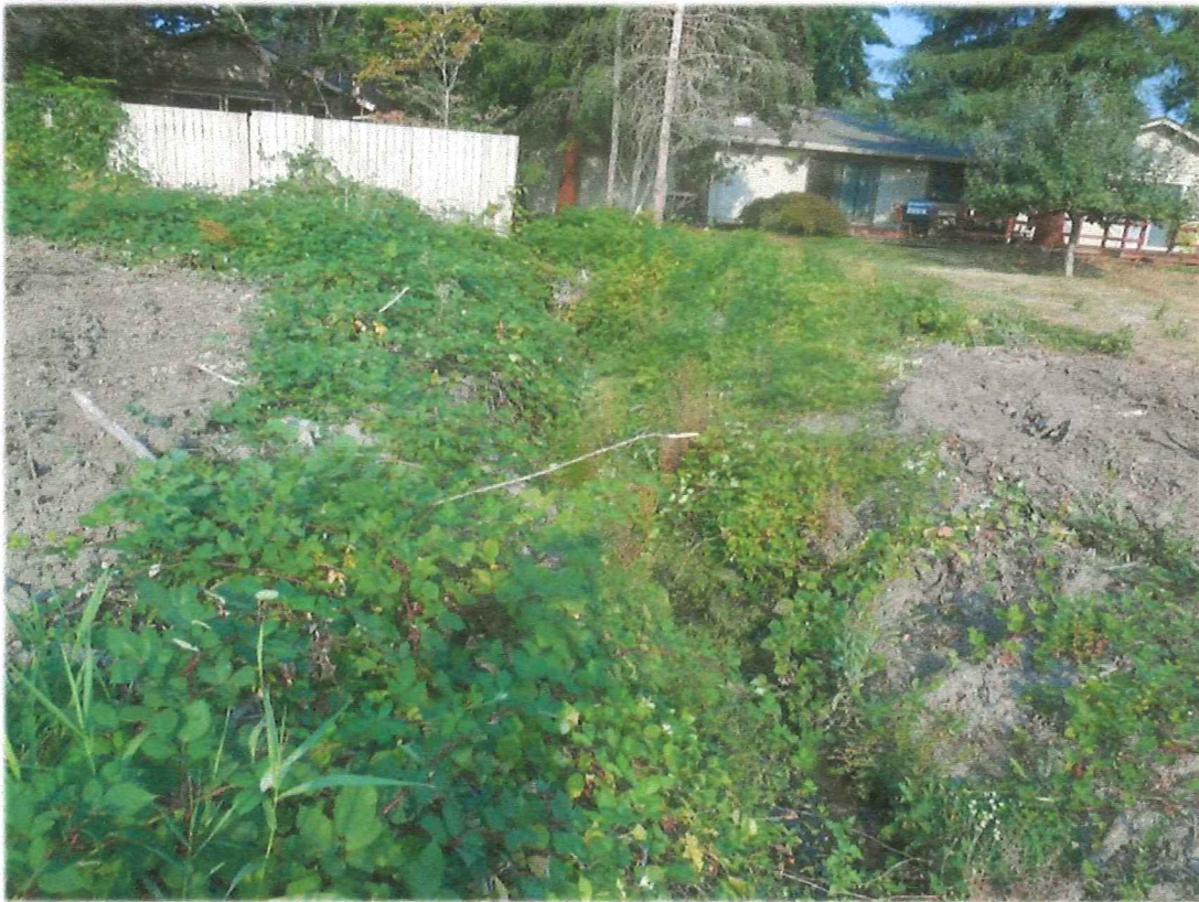
Photo Point 2. At western extent of drainage, Facing west.
