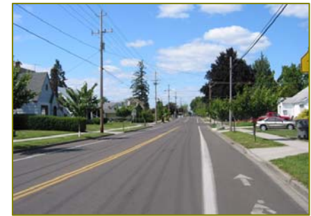
Recently Reconstructed Evans St
