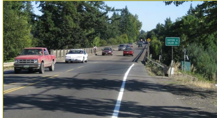
Yamhill River Bridge
