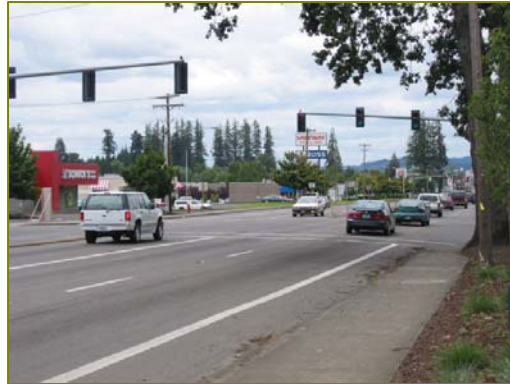
Traffic Signal on Hwy 99W at Lafayette
