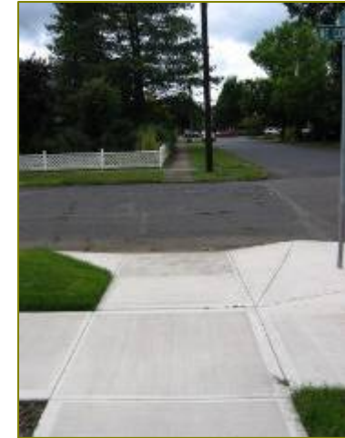
Perpendicular Curb Ramp
