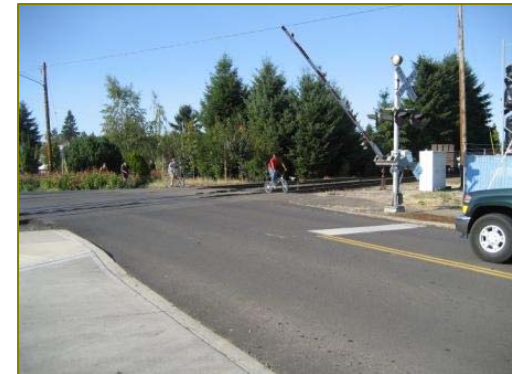
Missing Sidewalk at 8 th Street
