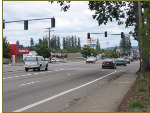
Traffic Signal on Hwy 99W at Lafayette
