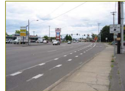
Bike Lane on Highway 99W
