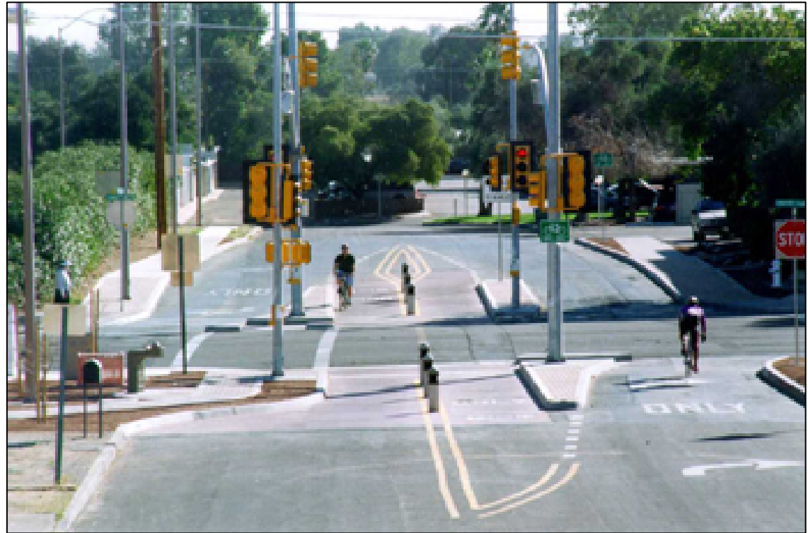
Allowing for Bicycle Access
