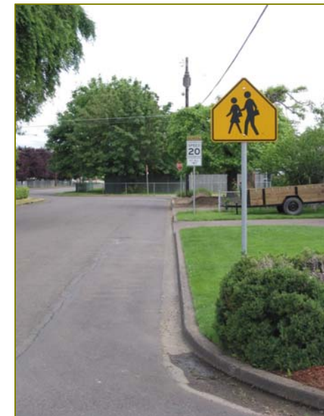
Missing Sidewalk in a School Zone
