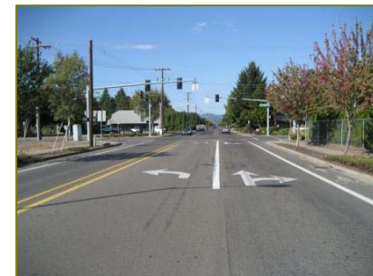
Bike Lane on Baker Creek Rd
