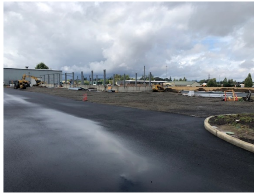
Phase 2-Building C Under Construction
