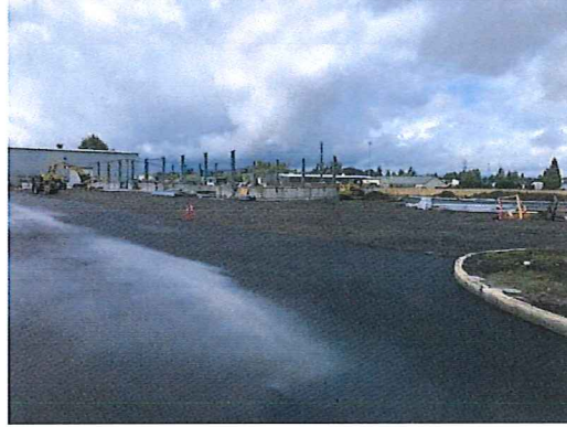
Phase 2-Building C Under Construction
