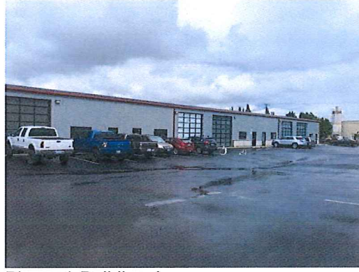
Phase 1-Building A
