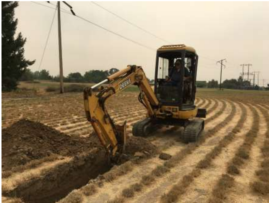
Test Pit TP-8, Facing South
