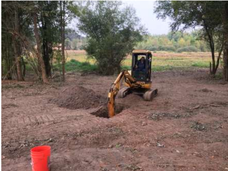
Test Pit TP-2, North-Central Portion of Site, in Wetland Area
