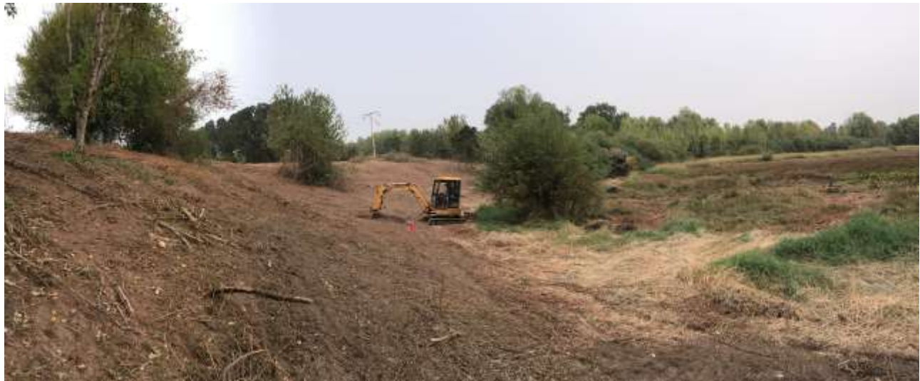
Facing North, Test Pit TP-9
