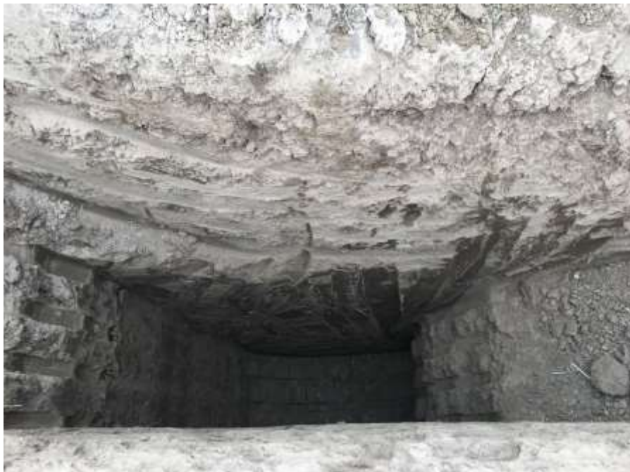
Test Pit TP-1
