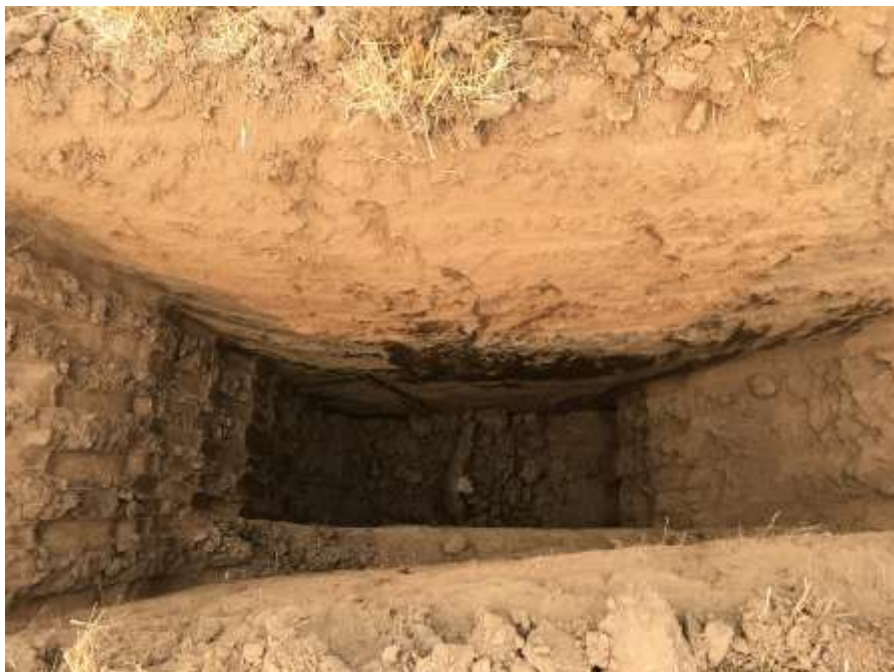
Test Pit TP-5
