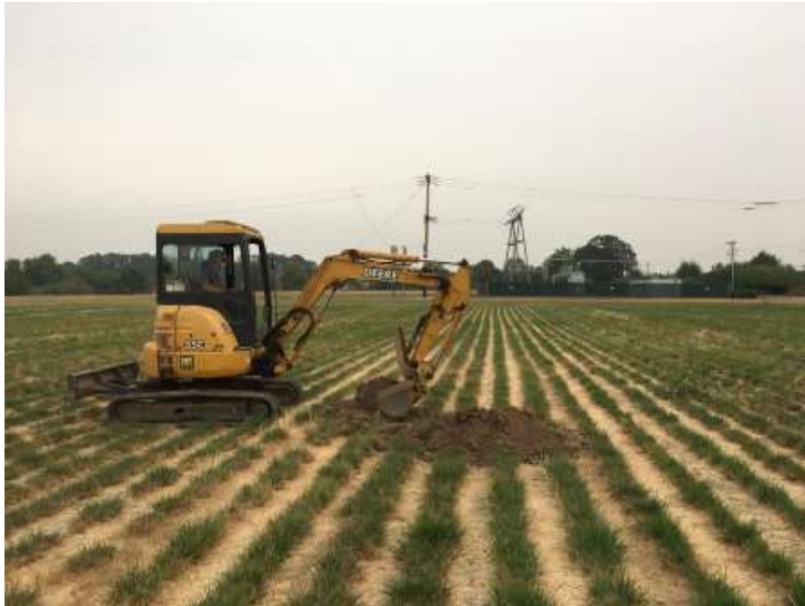
Test Pit TP-15, Facing South
