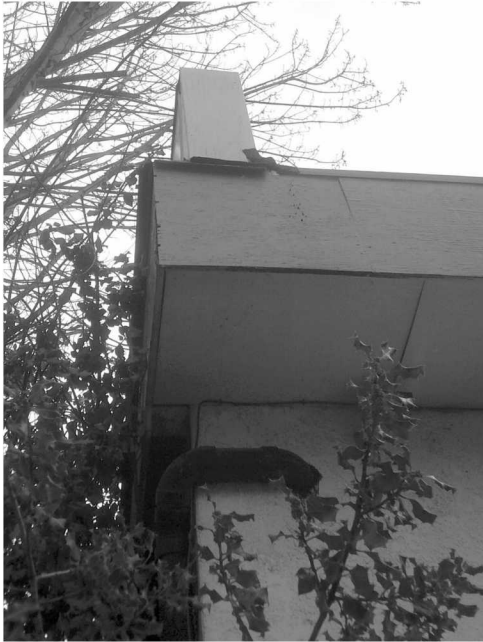
NW corner. Existing soffit and parapet wall.
