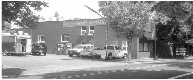
GVB west wall (on Hidalgo property line) and at Third St.
