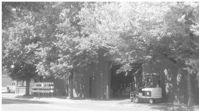
GVB wall at Third St, note overhead door, bays with no windows.
