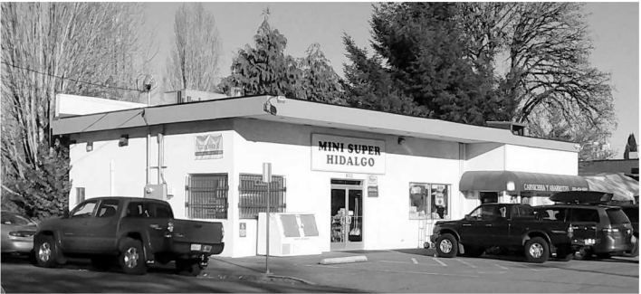
SW building corner, owner wants to enclose area under existing roof overhang
