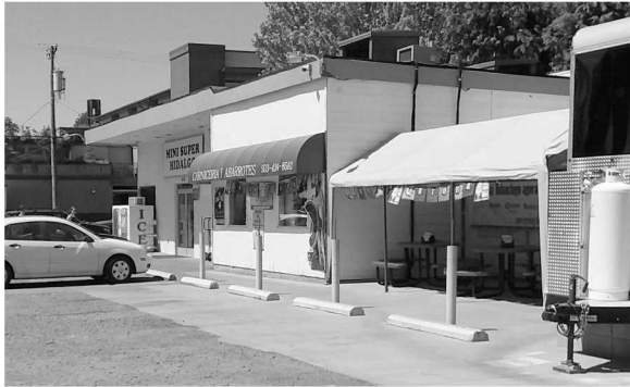
SE building corner, existing awnings to be removed.
