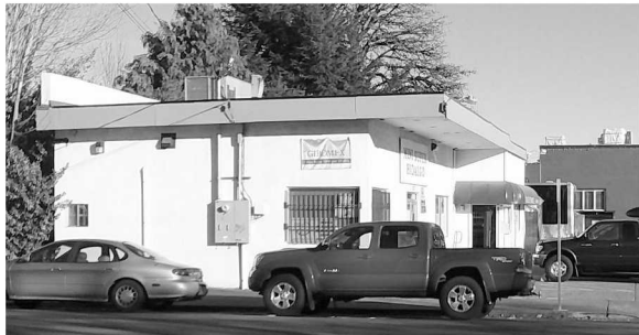
West wall, along Irvine St. Note overhead electrical service.
