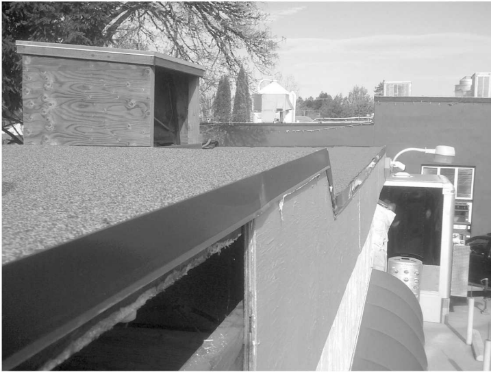
Roof looking east towards step down to wood framed addition
