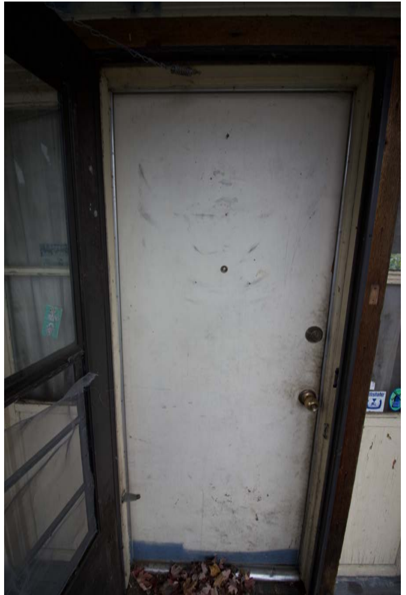
Replaced front door
