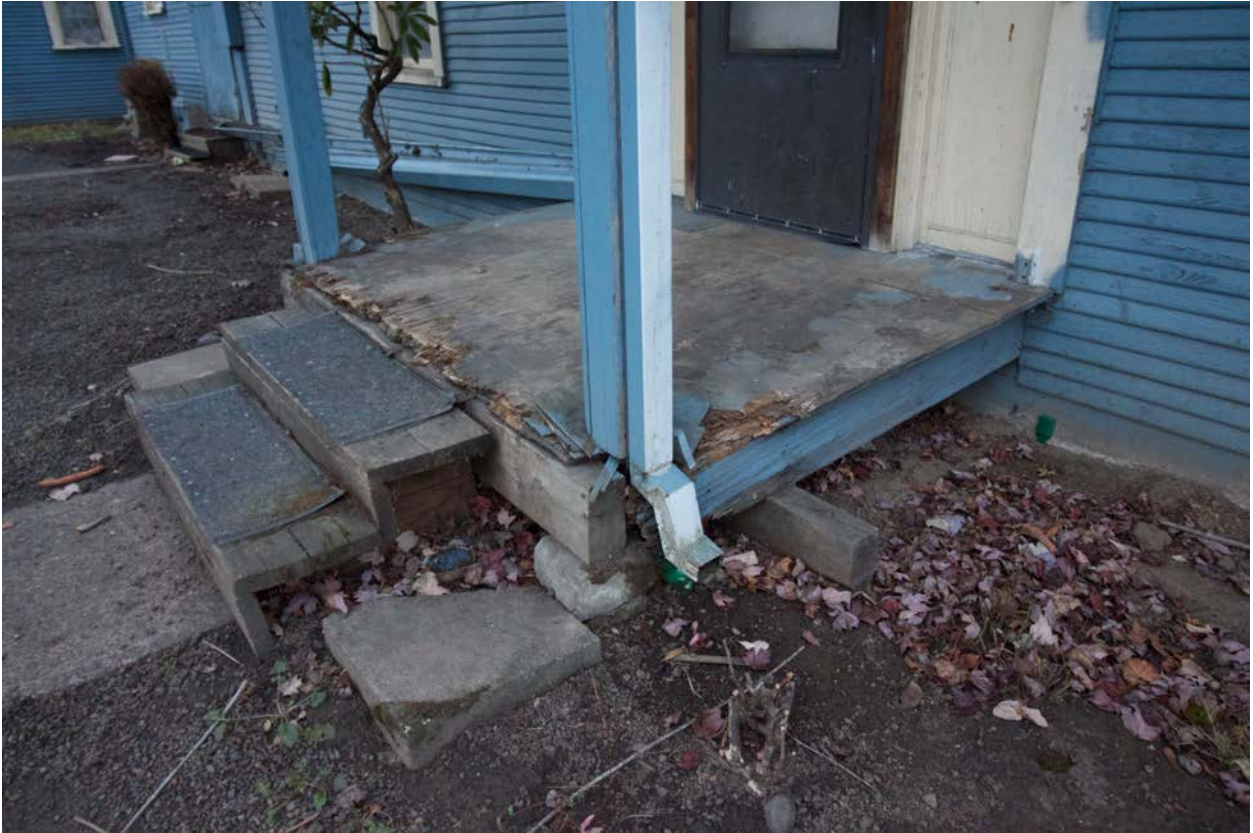
Current porch condition (West entry to Irvine)
