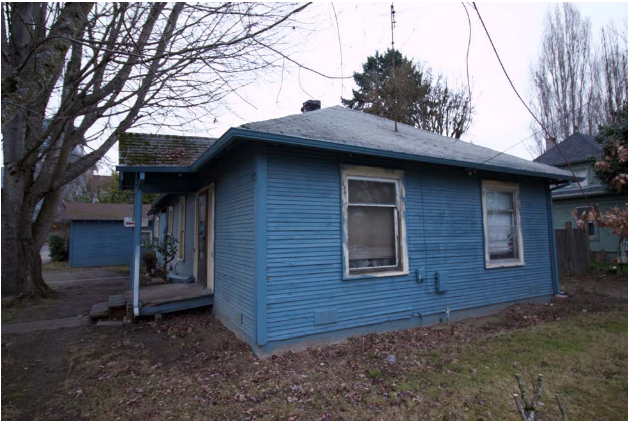
South side of house
