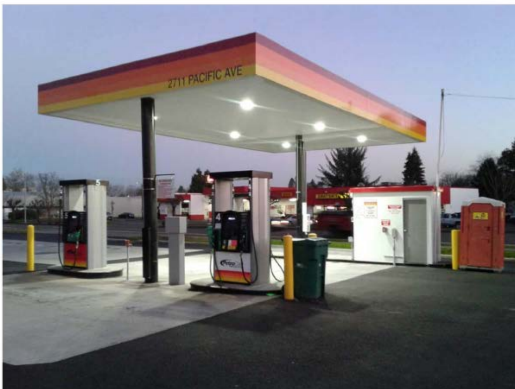
Photo No.1: This is a photo illustrating the canopy over the two fueling station dispensers.
