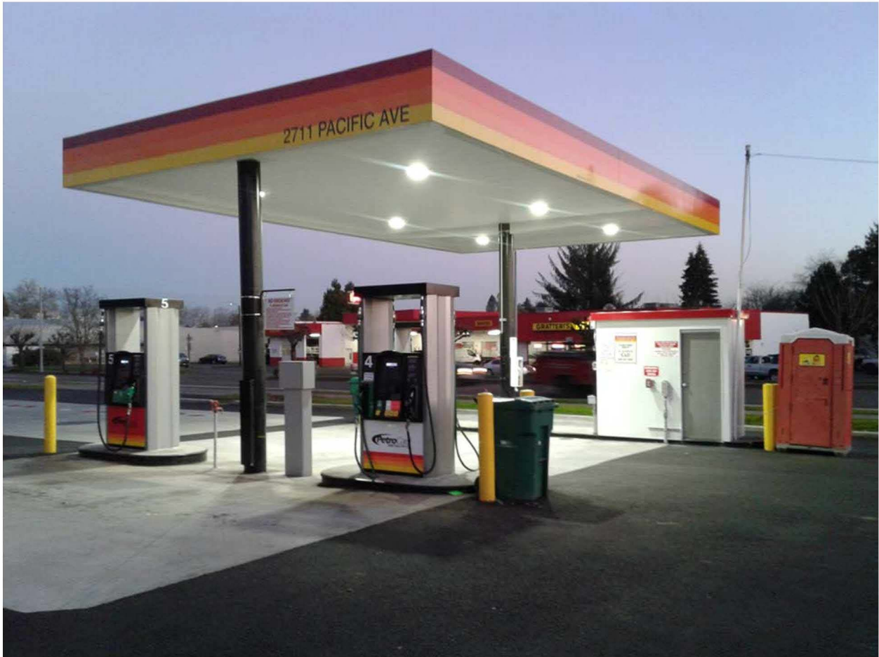
Photo No.1: This is a photo illustrating the canopy over the two fueling station dispensers.
