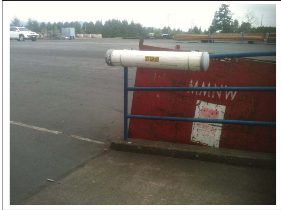
Catch Basin Cover near Catch Basin in Freight Ramp Area
