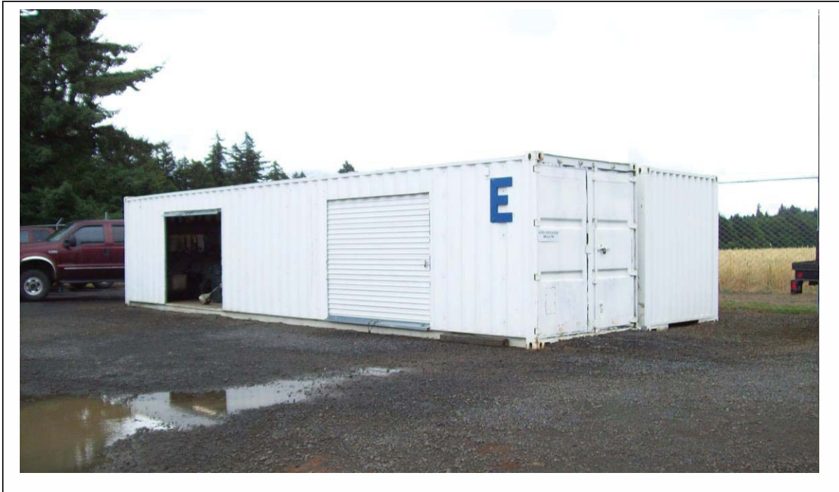
Conex Building for Maintenance Supplies
