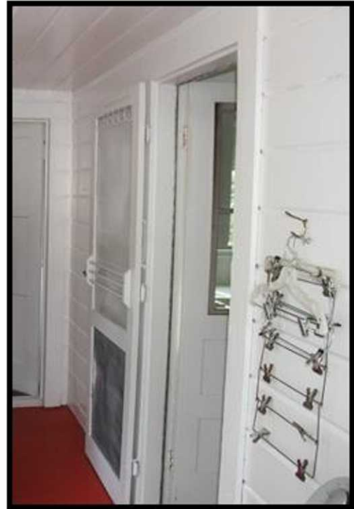
Figure 3: Screen door still in place within interior
