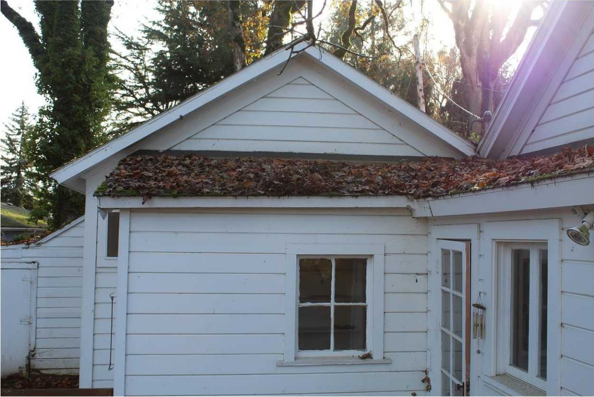
Figure 13: View from North of existing porch structures and roof line. Note also existing window trim.
