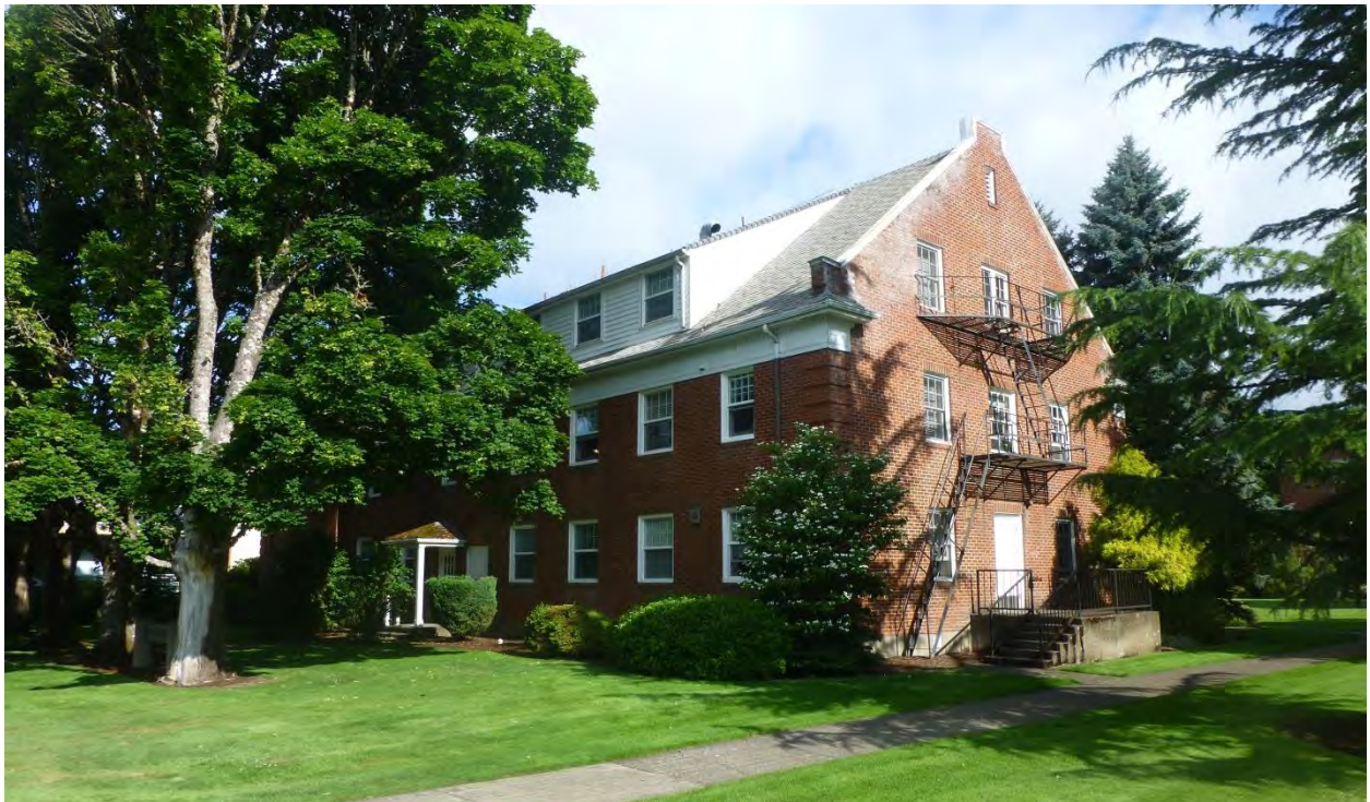
View of south elevation from Linfield Avenue looking to the northwest
