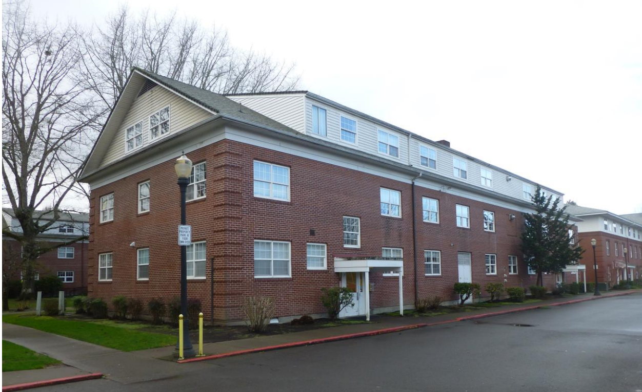
View of northeast elevation
