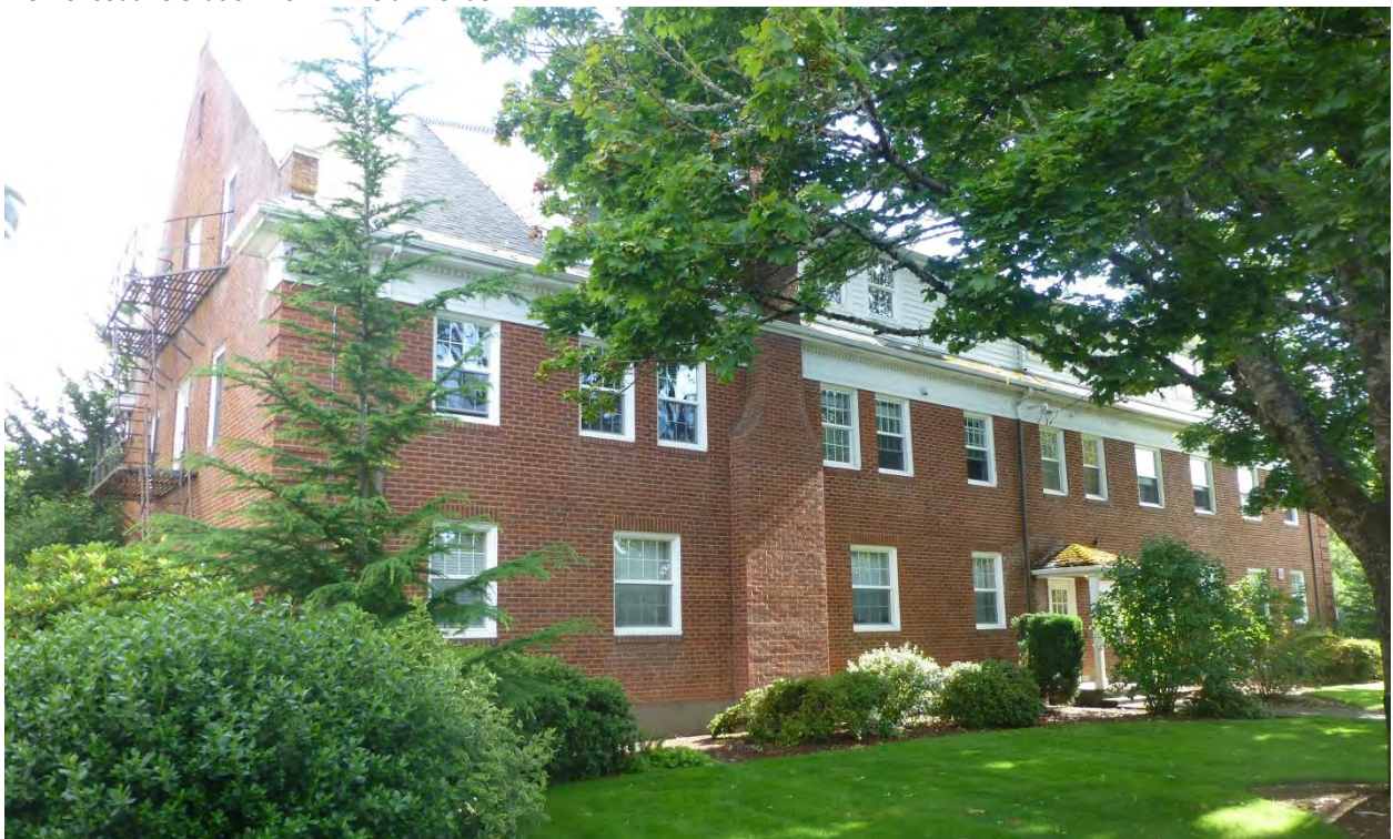
View of south elevation from Linfield Avenue looking to the northeast
