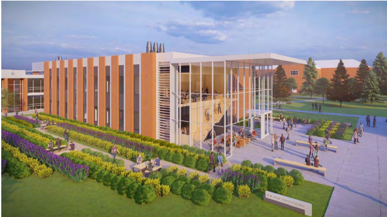
Overall view of Science Complex from the south east looking to the northwest
