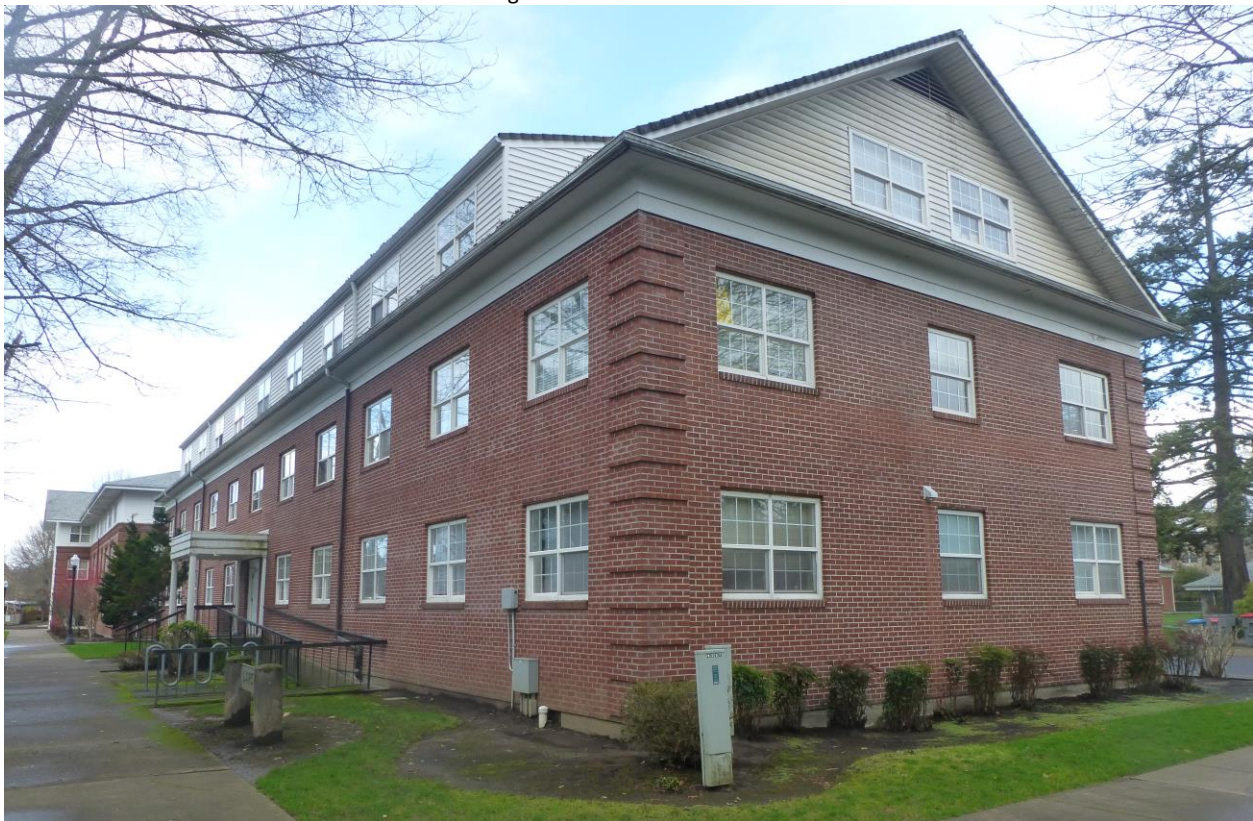
Detail view of northwest elevation
