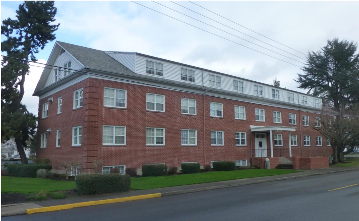
View from Linfield Avenue from the southwest looking to the northeast
