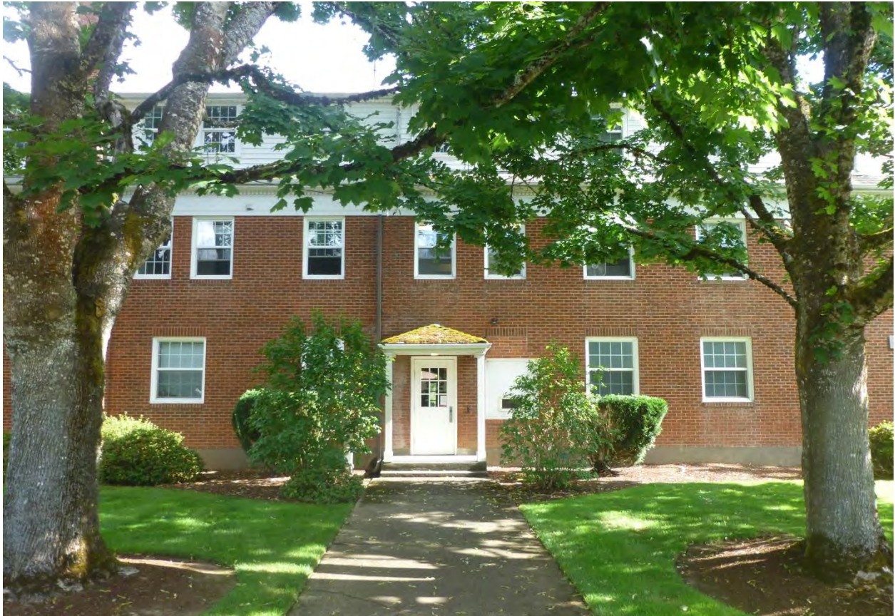
View of south elevation from Linfield Avenue
