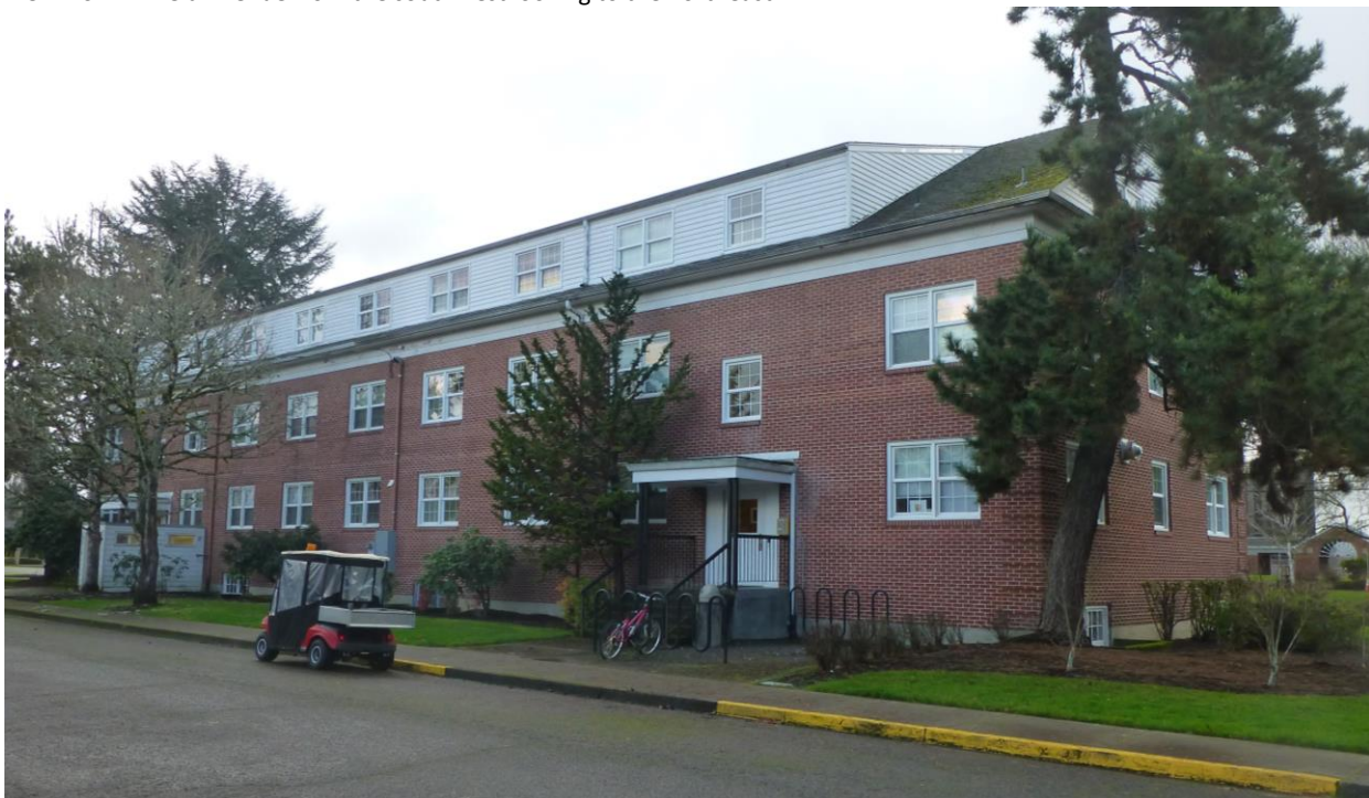
View of north elevation looking from the northwest
