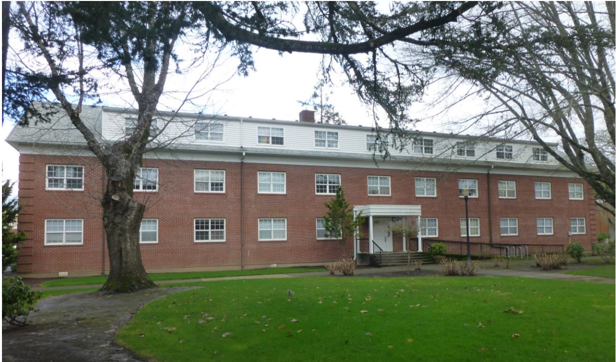
View of south elevation
