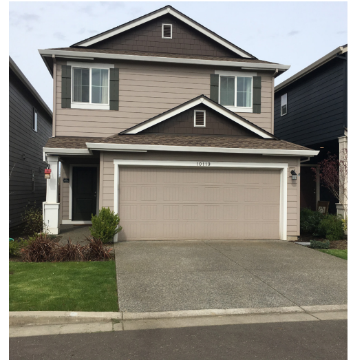
The garage and driveway dominate the façade, which does not meet the standards of a garage wall that is less than 50% of the overall width of the façade.
