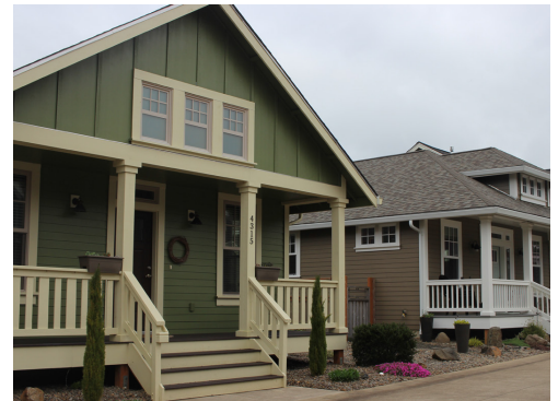
These homes have similar rooflines and porch elements, but they vary – one is gabled and one is hipped with a dormer making them distinct from one another.
