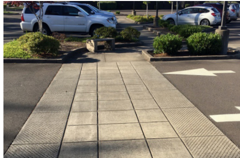
Example of a parking lot through connection
