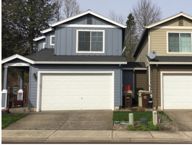
Driveway spacing does not provide enough space for a street tree or on-street parking.
