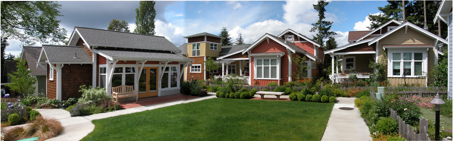
Cottages with layers of open space from private porches to common shared open space.
