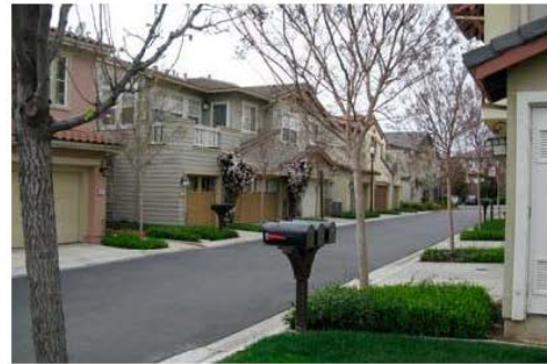
RECOMMENDED - Private streets should be lined with accent trees and planters to help soften the appearance of multiple garage doors.
