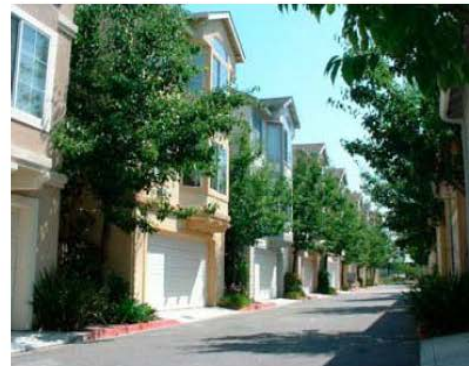
RECOMMENDED - Auto courts should be lined with accent trees and planters to help soften the appearance of multiple garage doors.
