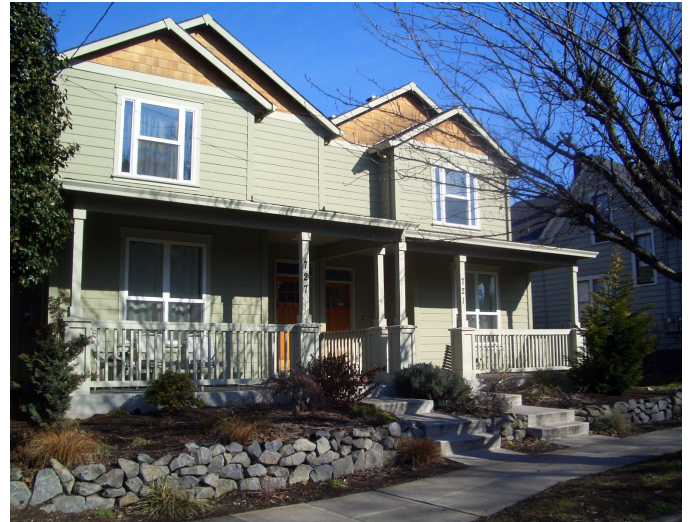
A porch railing separates entries and provides privacy to each unit, while creating a cohesive porch across the front.
