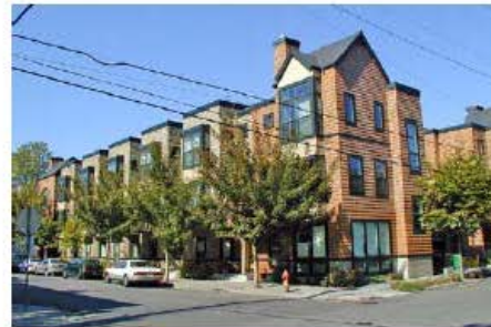
RECOMMENDED - Taller massing defines building features such as corners that create building articulation to reduce monotony.
