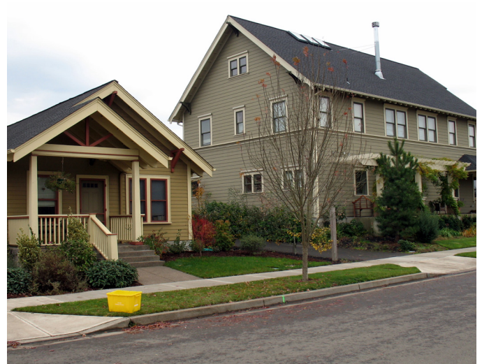
Changes in roof form or the incorporation of smaller scaled elements would improve the compatibility of the larger building adjacent to the bungalow.
