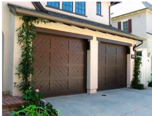
RECOMMENDED - High-quality wood or wood-like garage doors with decorative wood corbels and header.
