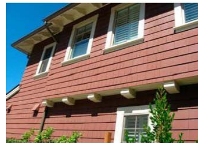
RECOMMENDED - High-quality detailing of exposed wood rafter tails, corbels, window surrounds and shingle siding.
