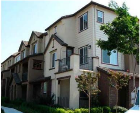
RECOMMENDED - Second and third floor massing and articulation should relate to ground floor.
