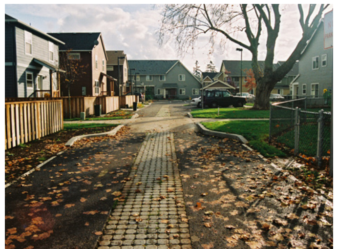
The curb physically and visually narrows the width of the alley. Permeable paving is built into the lowest point at the center to handle stormwater.
