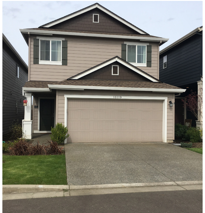
The garage and driveway dominate the façade, which does not meet the standards of a garage wall that is less than 50% of the overall width of the façade.
