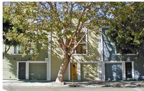
PROHIBITED - Building entries that are not prominent and appear secondary to the garage.
