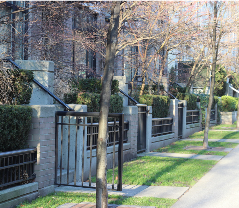
Landscaping, trees, and partially-open wall provide a transition with layers of privacy from the sidewalk edge to the apartment building.
