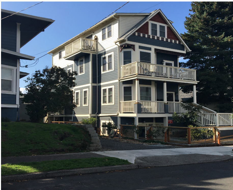
The scale and form of this plex fit with the surrounding context.
