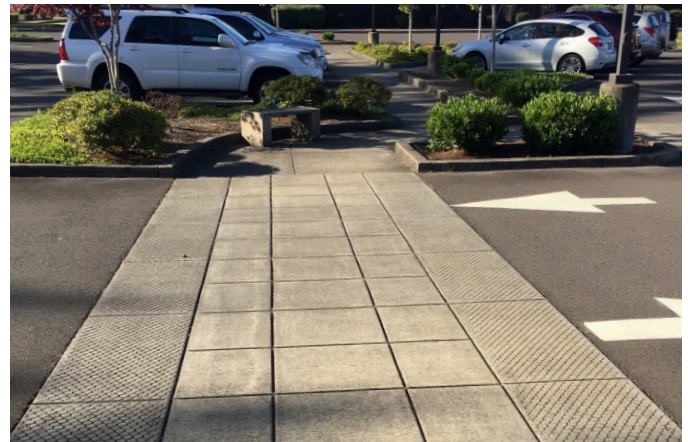
Example of a parking lot through connection
