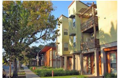
RECOMMENDED - Trellis and column material and proportions should be designed compatibly with project architecture to not appear applied to the building facade.
