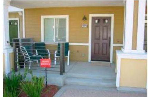
RECOMMENDED - Porches and patios should be raised 1'-3' above the grade of adjacent public streets or areas.
